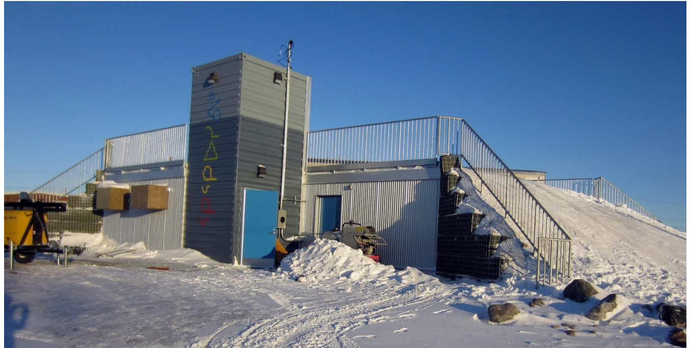
Figure 42: Arviat Community Freezer, Stantec Architects
