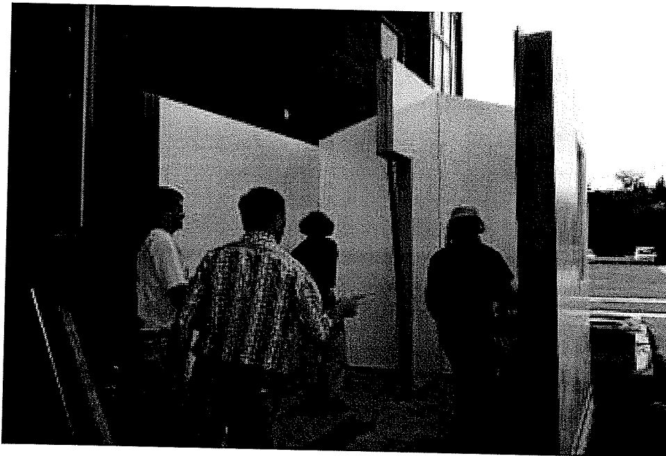
Photo 2: Installing the Partition Wall
