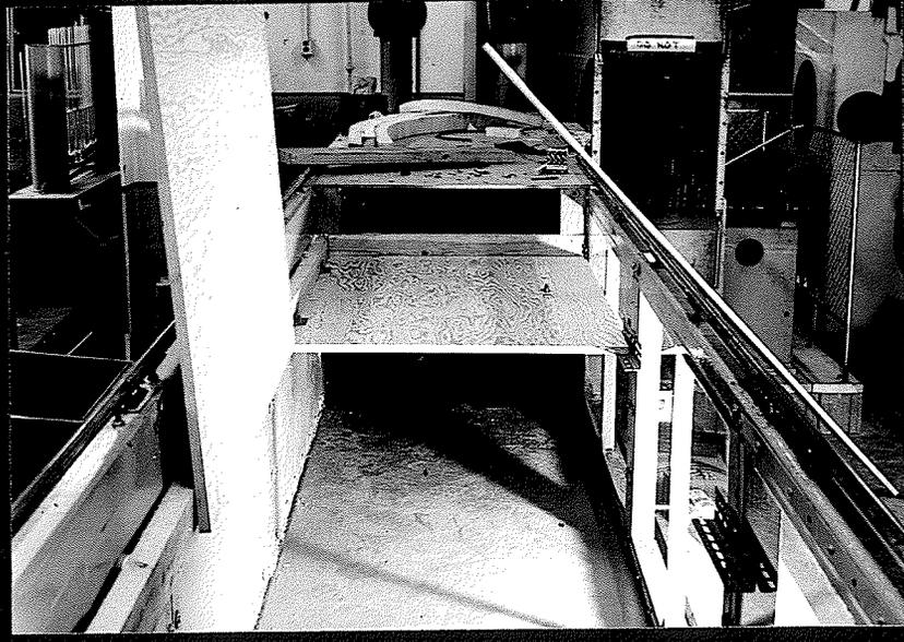
ILLUSTRATION XI: Installation of top panels of wind tunnel. The panels were opened as shown between tests for alterations in the wind tunnel. Small ports were cut in the panels for access during a test.
