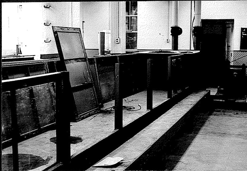
ILLUSTRATION X: Glass and steel side panels of hydraulic flume during construction. When completed, one side of the wind tunnel was entirely glass.
