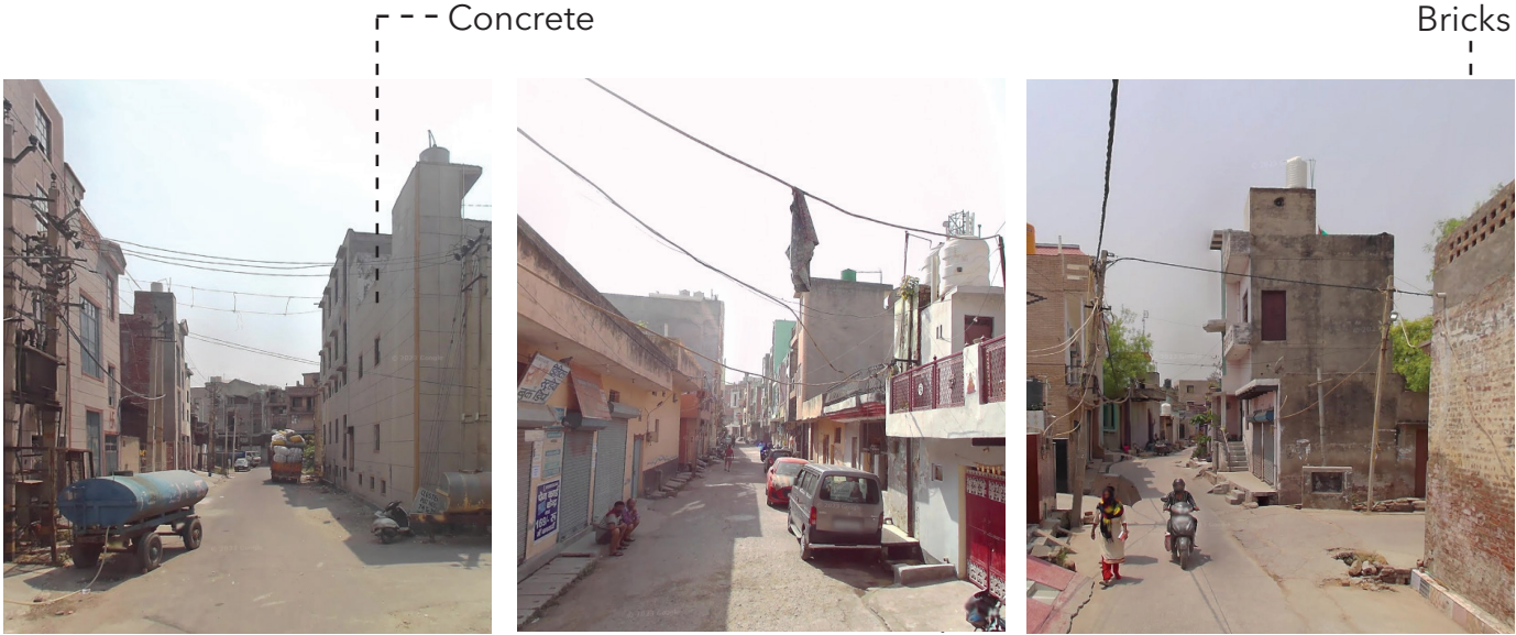
Fig.11. Delhi street images showing overdominance of impervious surfaces.
