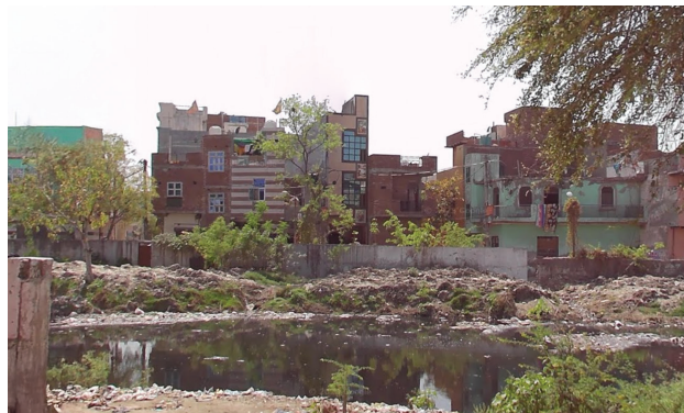
Fig.32. View of degraded Drain near the Nala Rd, Delhi.
