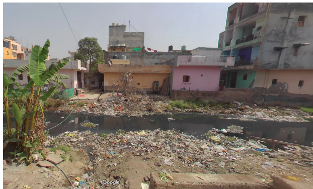
Fig.33. View of degraded Drain near the Bhagat Singh Rd, Delhi.
