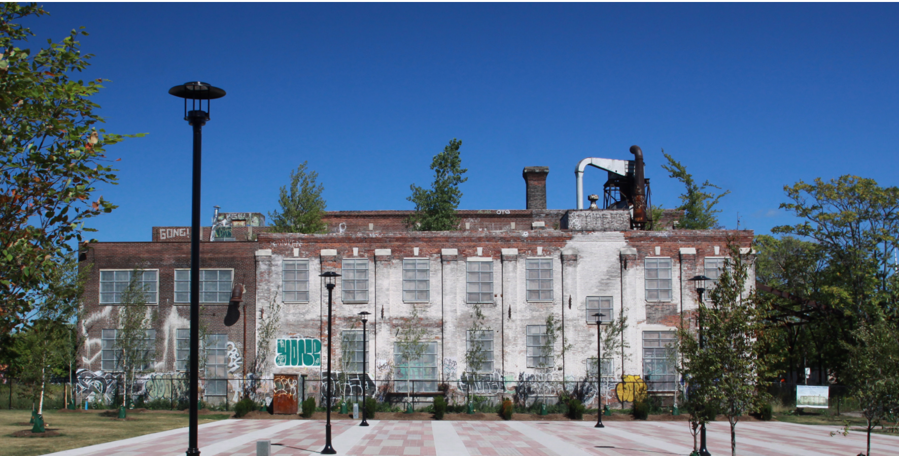
FIGURE 25 - 40 WABASH AVE WEST FACADE
