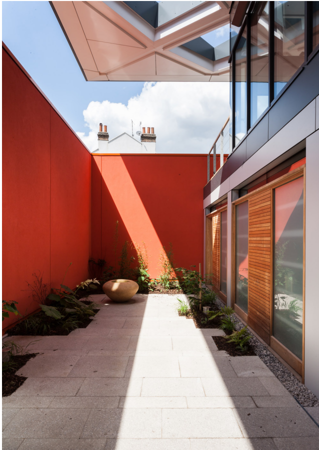
FIGURE 12 - MAGGIE'S WEST LONDON EXTERIOR WALL WRAPPING AROUND BUILDING
