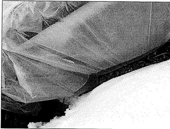
Figure 32 Water in the headspace of the biofilter during the winter
