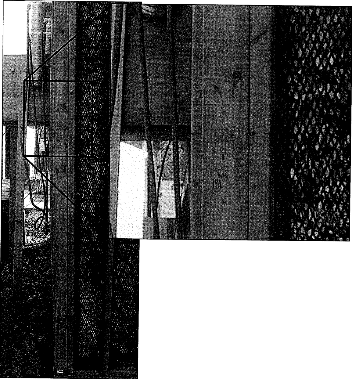
Figure 33 Biofilter wall creeping outwards
