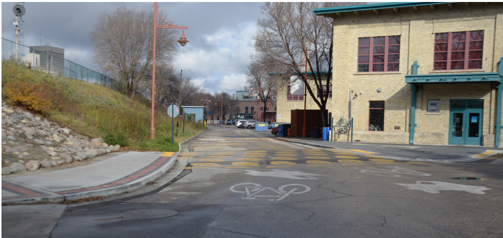
Figure 6: Raised Crosswalk from Phase 2 Before and After Construction (source: Google Earth)
