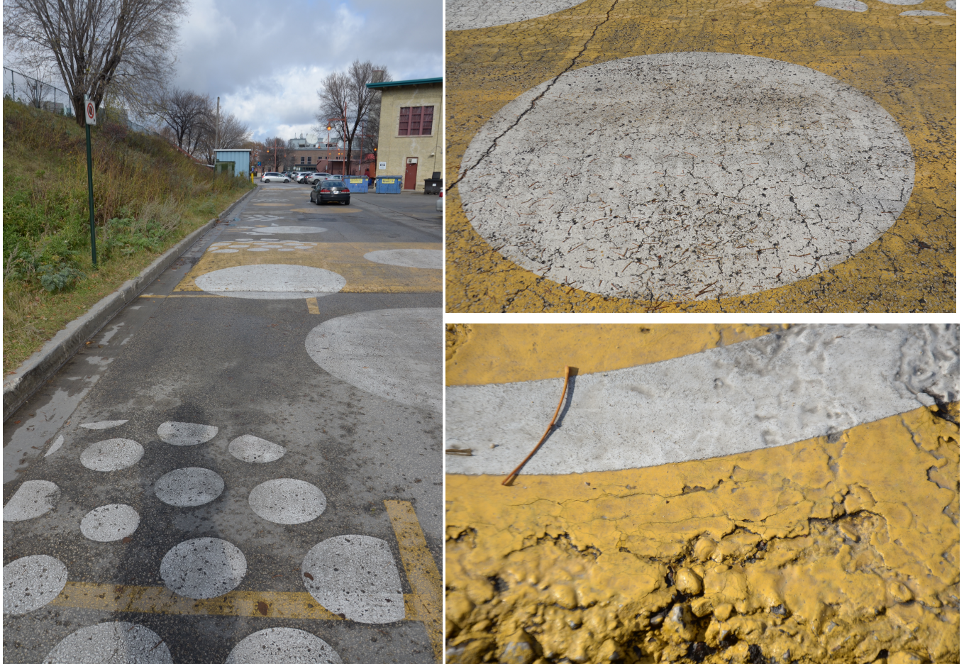
Figure 15: Photographs from October 2016
