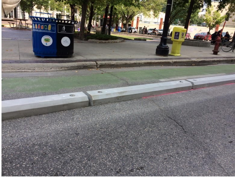
Figure 22: Bannatyne Avenue Adjustable Bike Curb Pilot (City of Winnipeg, 2017)
