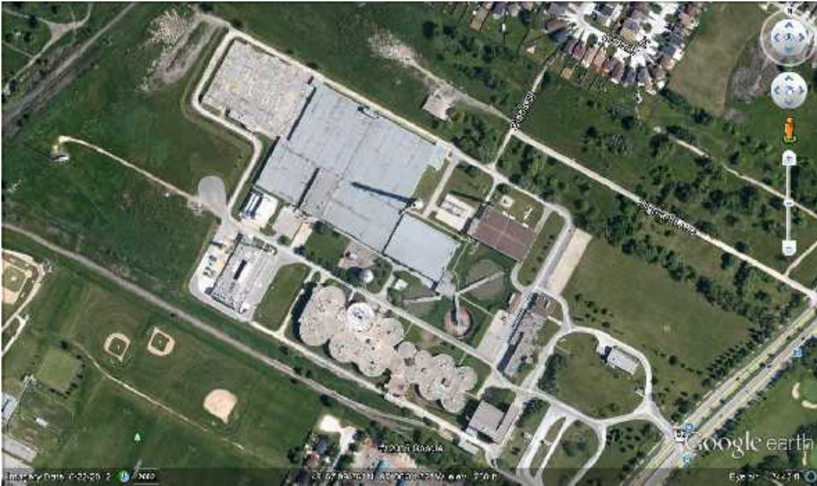
Figure 1.7 The Winnipeg North End Water Pollution Control centre. Image taken from Google Earth (2015).
