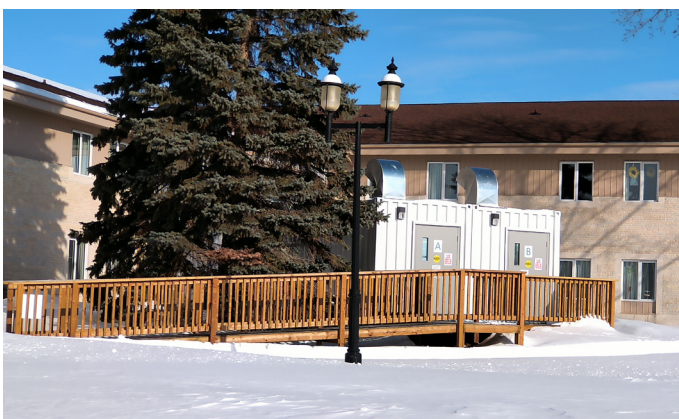
Figure 4: These shelters were located outside a small-town personal care home (171 beds).
