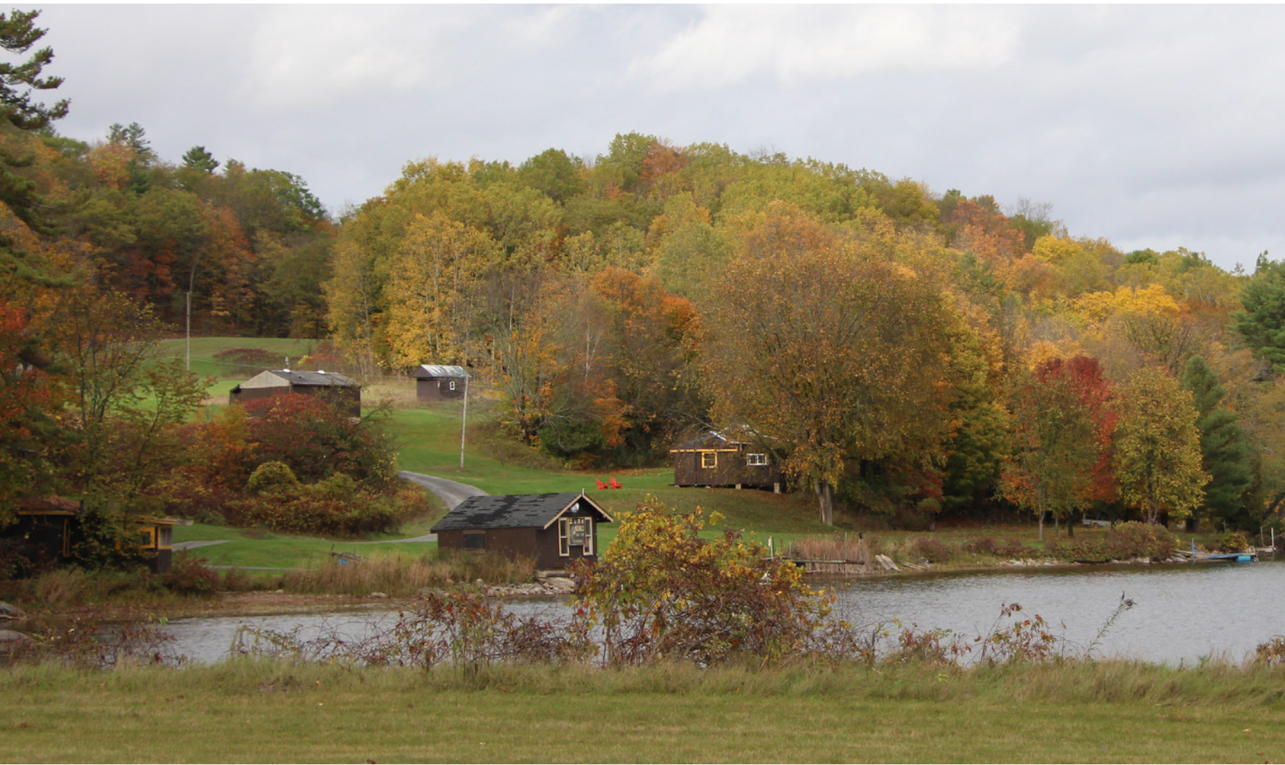
Figure 18. TimBer Landing depicting existing conditions along the shoreline
