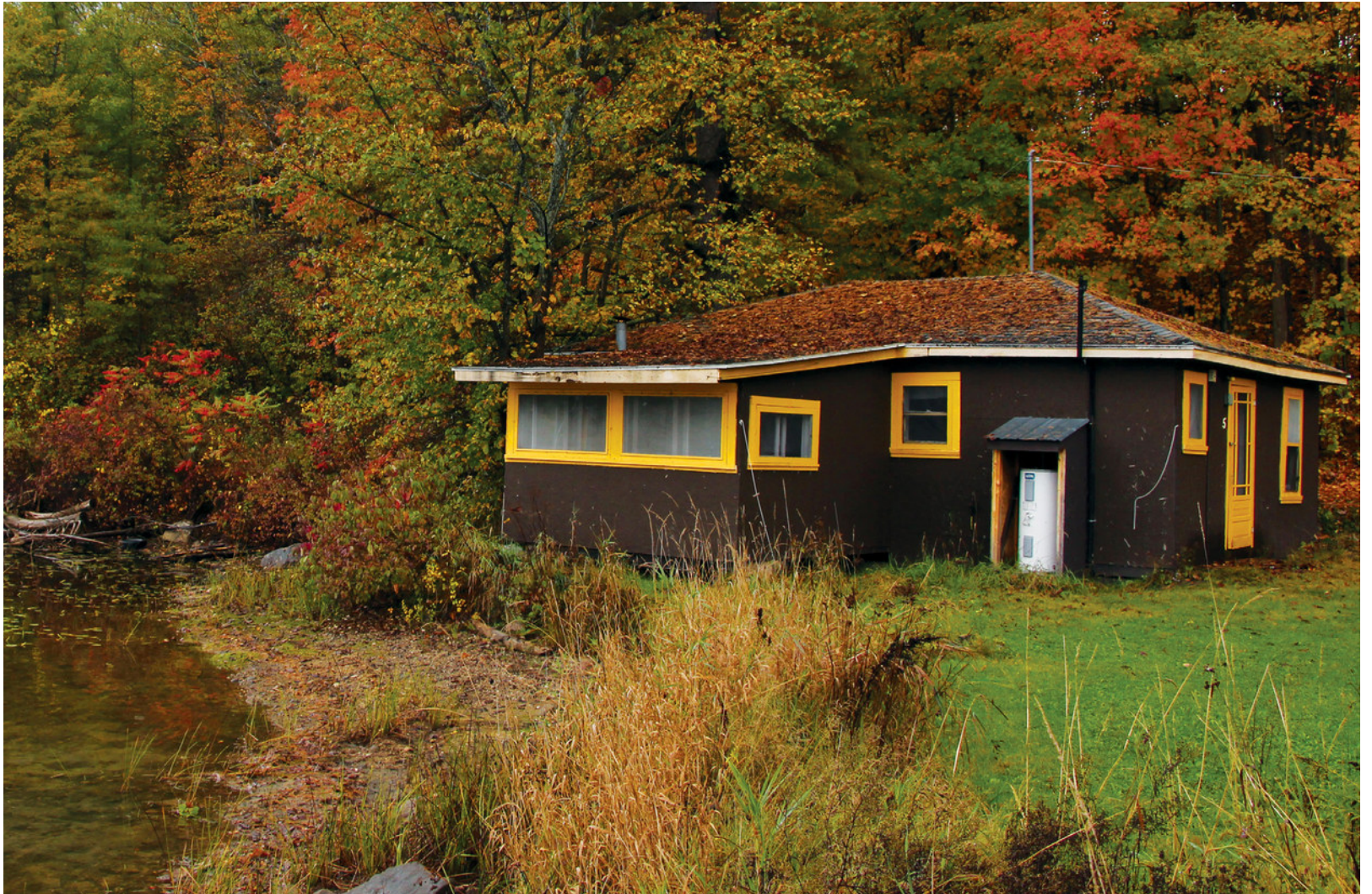
Figure 87. One of five cabins with this one being built right at the shoreline
