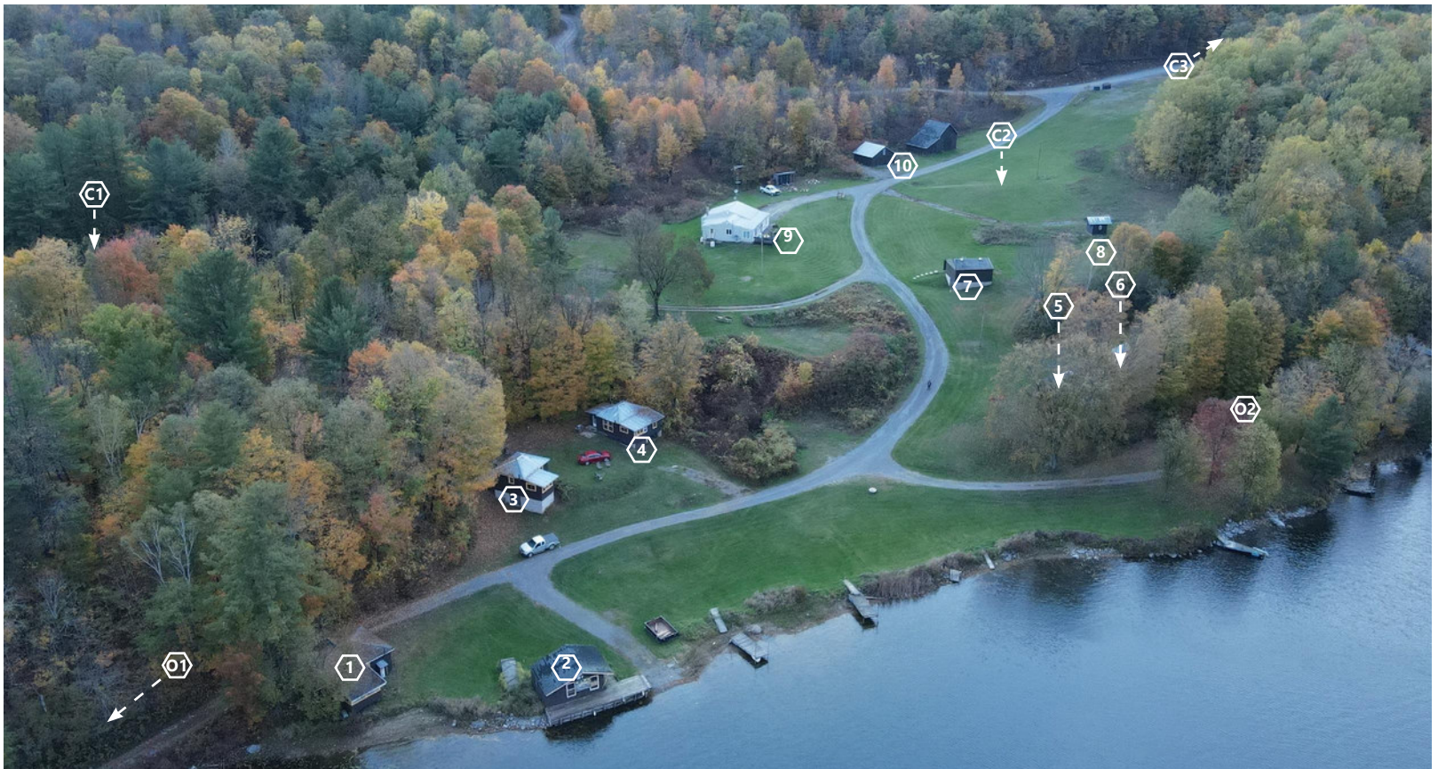
Figure 30. View of the existing structures on site
