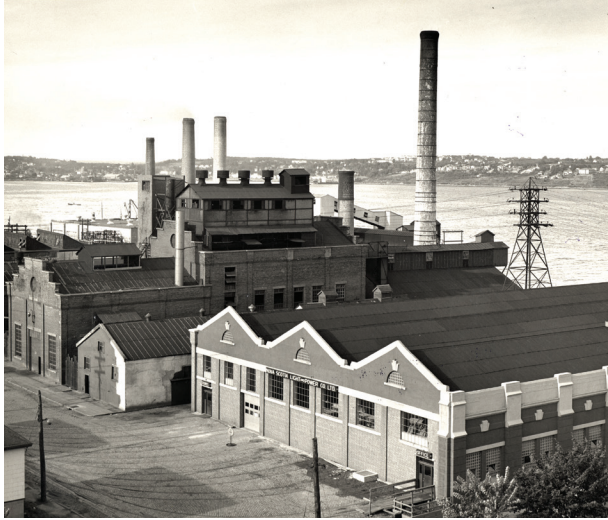
Figure 6.08 Nova Scotia Light and Power Company, Halifax, Nova Scotia.
