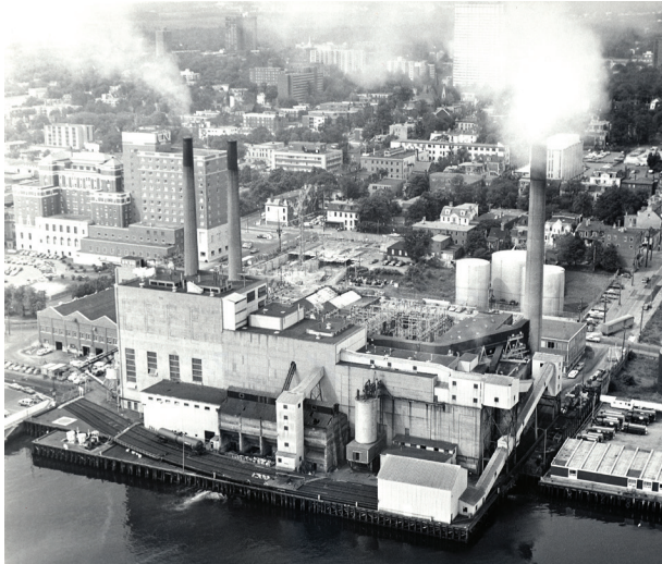
Figure 6.10 Nova Scotia Light and Power Company, Halifax, Nova Scotia.
