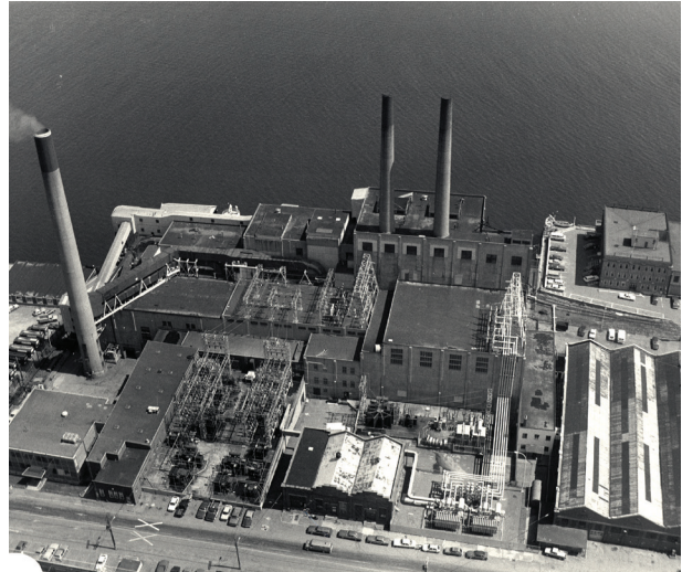
Figure 6.11 Nova Scotia Light and Power Company, Halifax, Nova Scotia.
