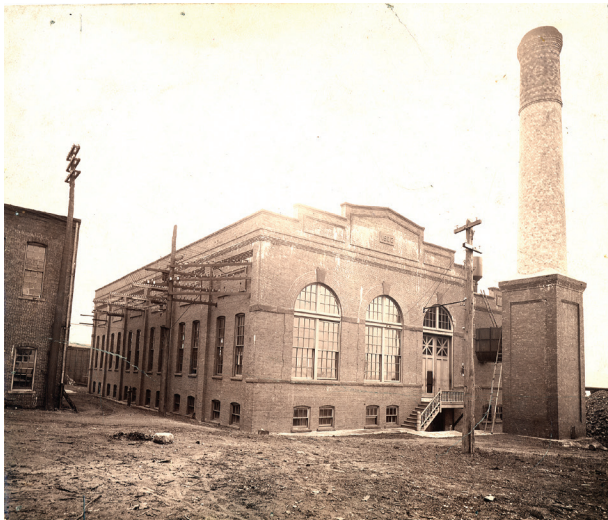
Figure 6.06 Nova Scotia Light and Power Company, Halifax, Nova Scotia.
