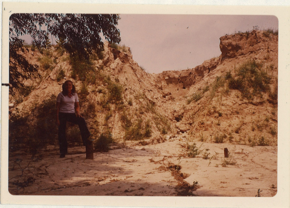
Photo #23: Sand material is particularly susceptible to erosion when exposed during a mining operation. In this picture, a property boundary fence is almost covered over.
