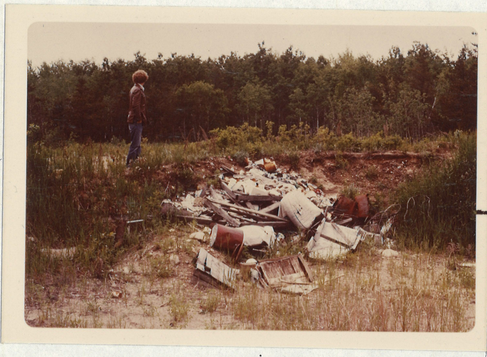
Photo #24: Abandoned or unused pits seem to attract abuse as convenient garbage disposal sites. This type of post mining land use is often the least desirable since it may lead to ground water contamination.
