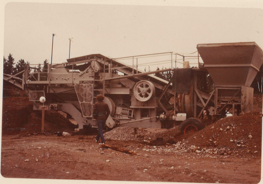
Photo #7: A portable crusher, used to break rock into specified sizes.
