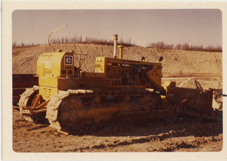
Photo #25: The bulldozer is commonly used in Manitoba for final grading of depleted pits, in compliance with government regulations. The resultant slopes, as seen in the background, reflect the machines performance in their gradient (usually 18 degrees) and form.
