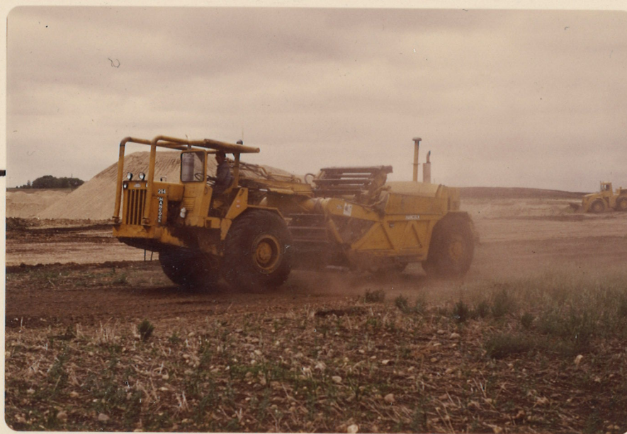
Photo #4: Scrapers are the most effective machine for stripping large areas.
