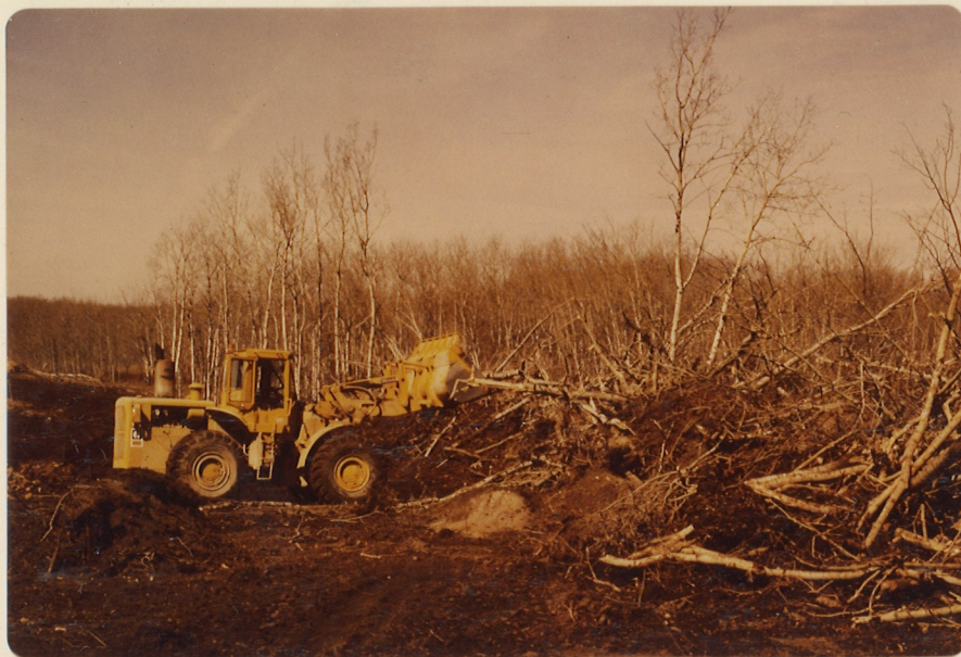
Photo #3: Loaders are commonly used to simultaneously clear and strip, with unfortunate consequences.
