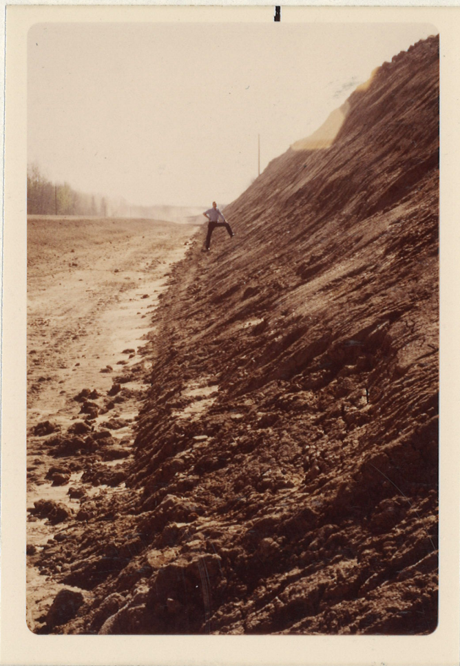
Photo #21: This recently formed slope, at 41 degrees, is virtually untraversable. It is highly susceptible to erosion and visually incongruent with the adjoining landscape.
