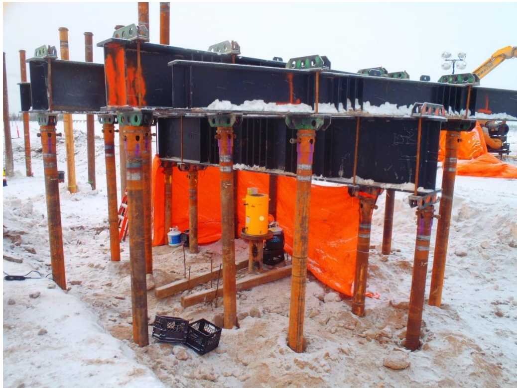
Figure 3.3 - Typical Load Test Set Up
