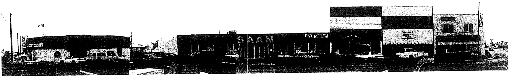
Figure 13. West side of Main Street streetscape 3
