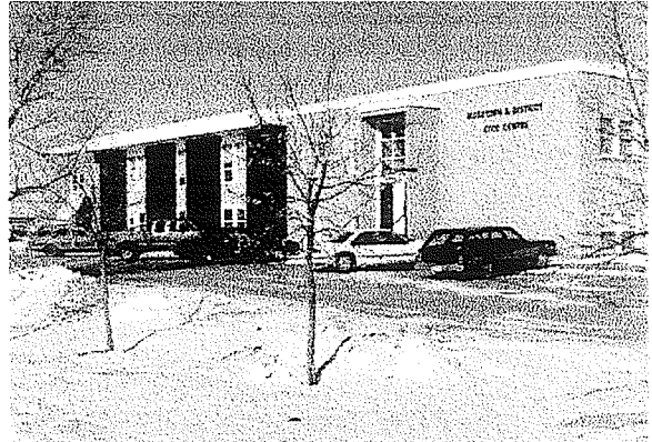
Figure 37. Rosetown & District Civic Centre
