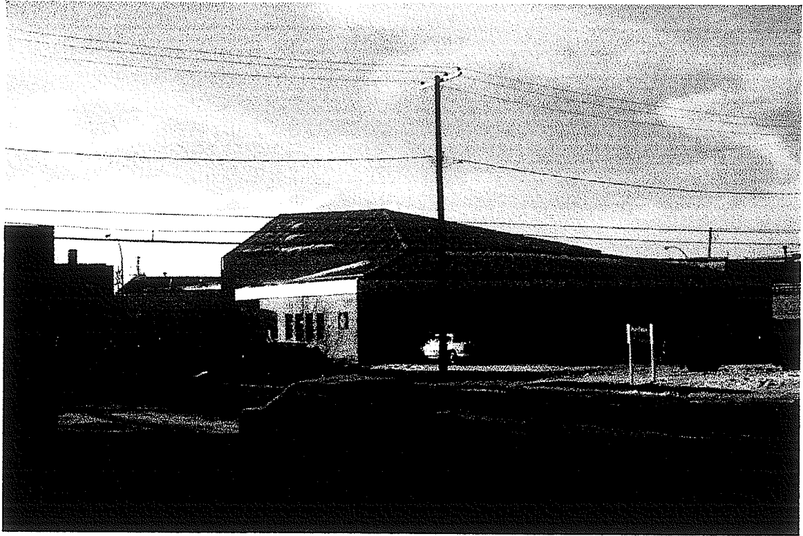
Figure 108. Exterior photograph 18, RDCU building, alley side
