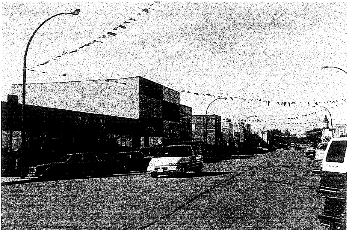
Figure 95. Exterior photograph 5, Main Street, northward
