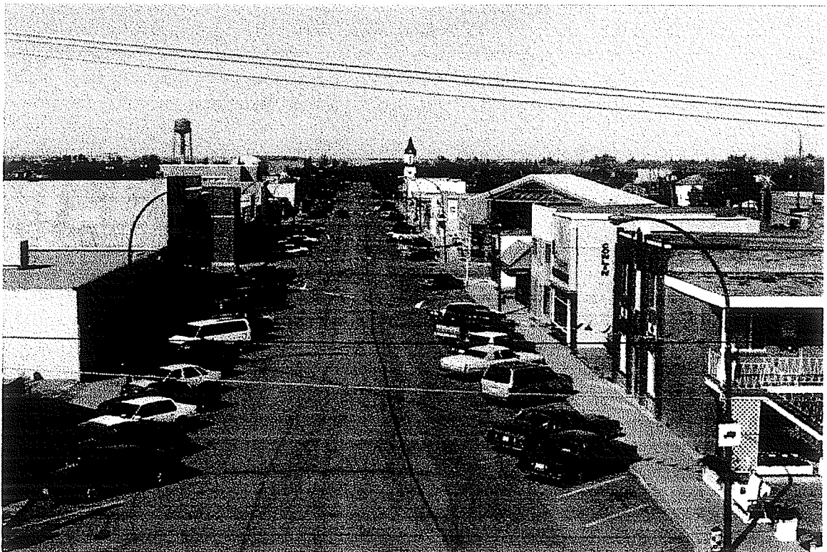
Figure 97. Exterior photograph 7, Main Street, northward
