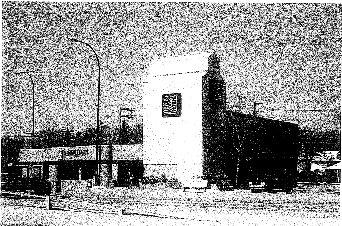
Figure 88. Royal Bank, Pembina Highway, Winnipeg, Manitoba
