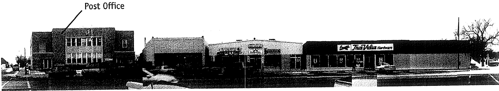
Figure 11. West side of Main Street streetscape 1
