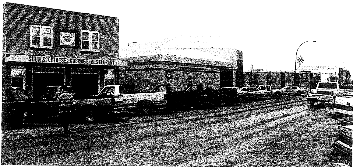
Figure 101. Exterior photograph 11, panorama featuring RDCU building
