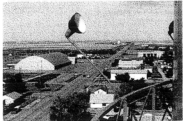
Figure 18. Highway 4 from the water tower, northward
