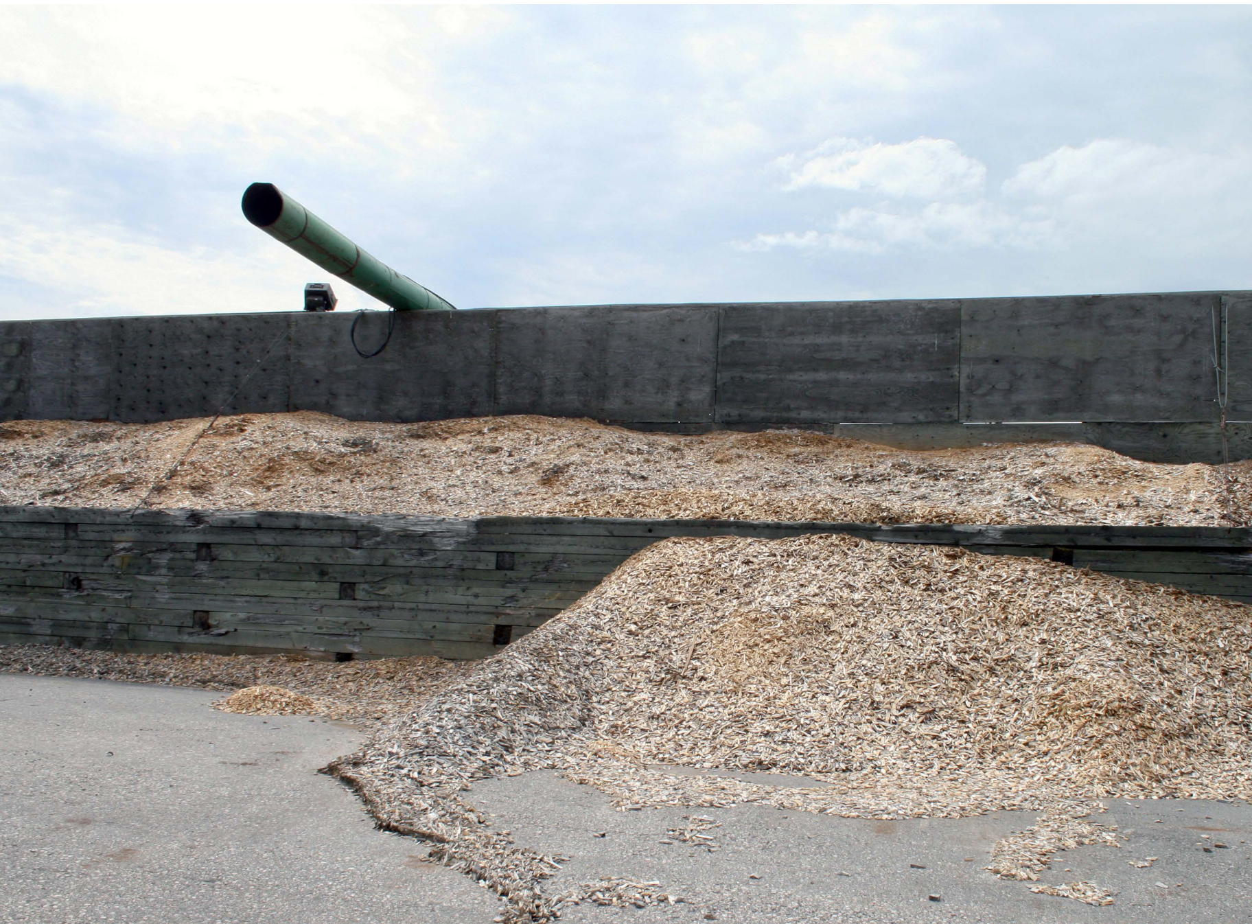
FIG. 5.36 Volume of woodwaste on site in perspective
