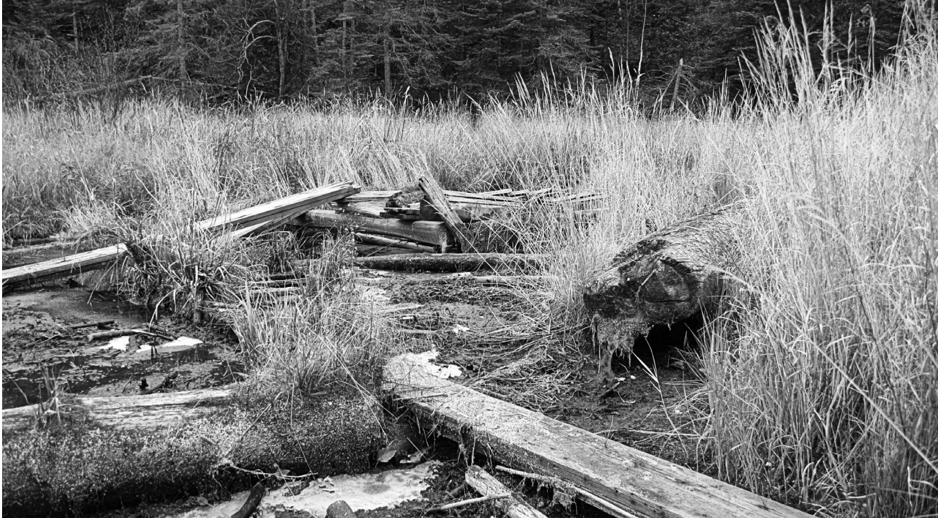
FIG. 4.19 Residual logs and lumber on Cameron Bay shore
