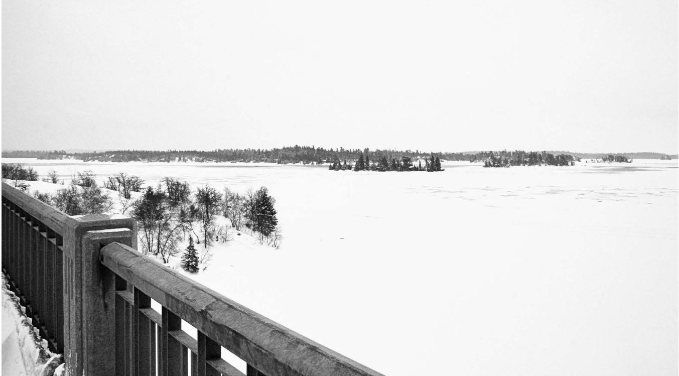
FIG. 5.4 View east of Lake of the Woods from highway
