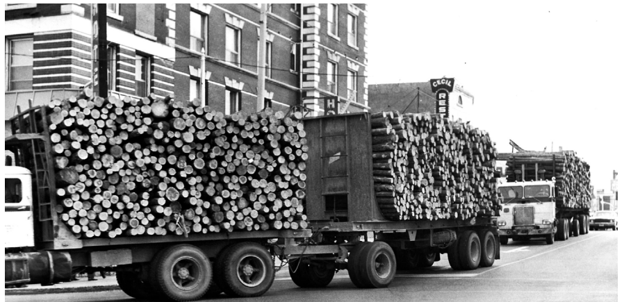
FIG. 3.11 bottom, log trucks at Kenricia Corner (Main St. and 2nd St. Intersection downtown)
