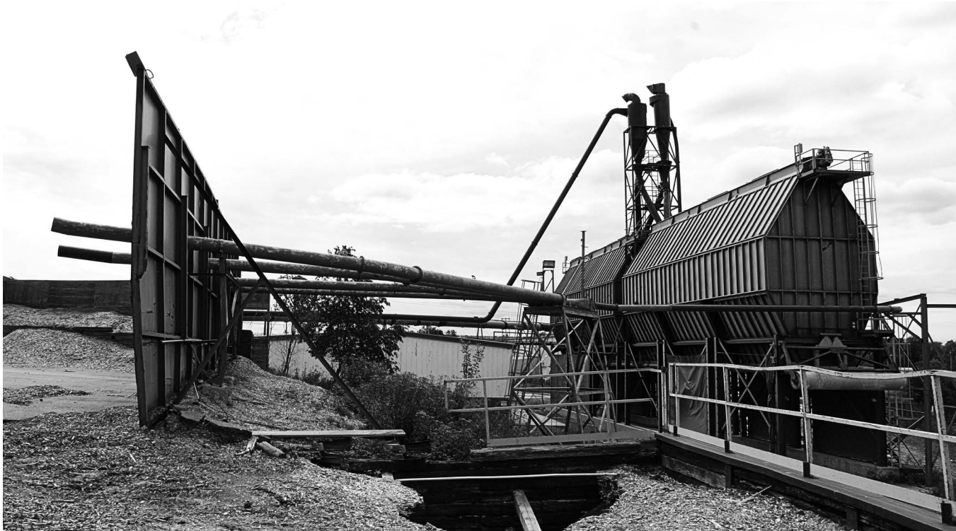
FIG. 5.37 View south of chip loader and woodwaste
