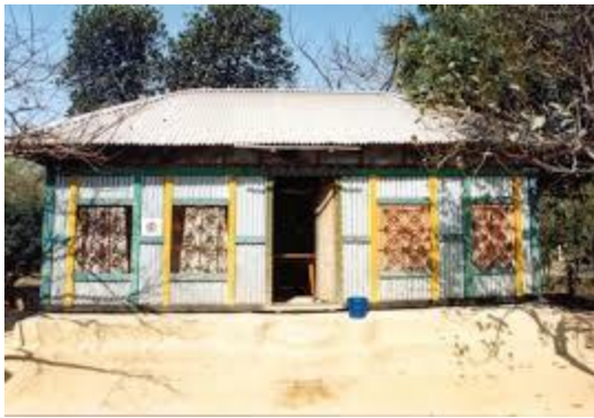
Figure 6 House with C.I. sheet walls and roof ( Source: World Habitat Awards, 1998 )
