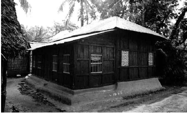
Figure 5: Timber house with C.I. sheet roof ( Source: Rashid, 2007 )
