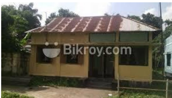
Figure 7: House with brick walls and C.I. sheet roof ( Source: bikroy.com, 2012 )
