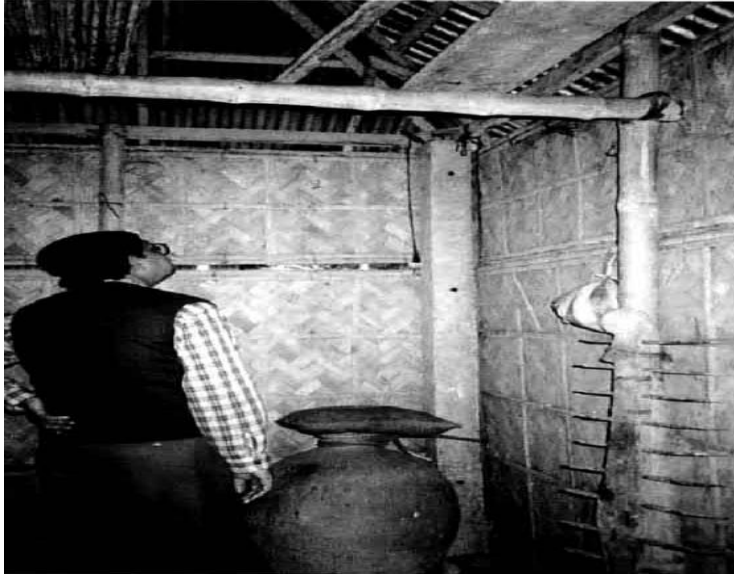
Fig 3: Bamboo mat wall with C.I. sheet roofing ( Source: Rashid, 2007 )
