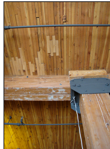
(Bottom Left) Figure 39 Remnants of the concrete that once covered the original timber columns and joists. Photograph by author (Bottom Right) Figure 40 Steel collars added by Nyygard to prevent further splitting of the timber columns. Photograph by author
