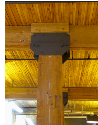
(Bottom Left) Figure 39 Remnants of the concrete that once covered the original timber columns and joists. Photograph by author (Bottom Right) Figure 40 Steel collars added by Nyygard to prevent further splitting of the timber columns. Photograph by author
