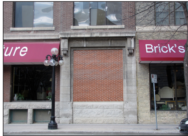
(Bottom Right) Figure 45 Previously used delivery access door along the south facade of 145 Market Ave. Photograph by author
