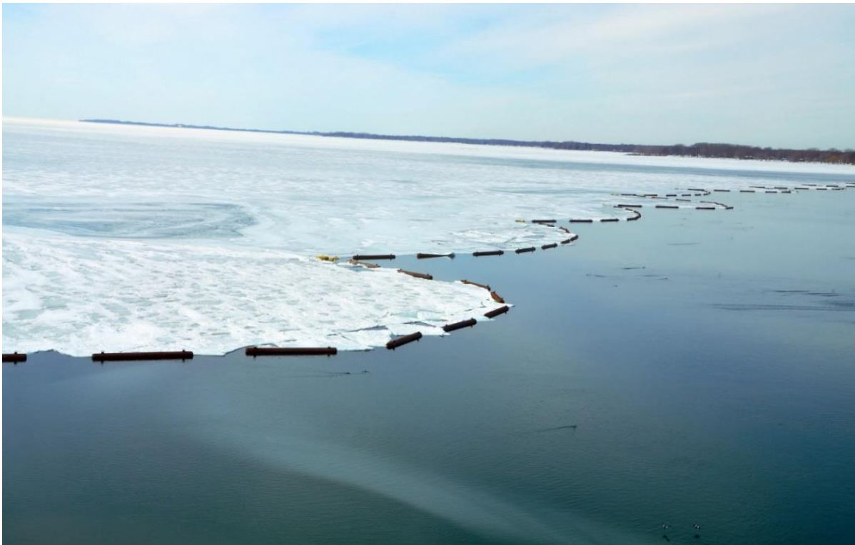
Figure 1.1. Pictures of (a) floating pontoons of booms in open water (Source: ODINBoom®) and (b) ice booms with upstream ice cover (Source: Ontario Power Generation).
