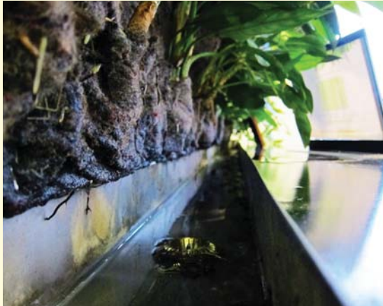
Figure 3.21: Felt Growing medium with water collection tray at bottom of hydroponic garden, Toronto.
