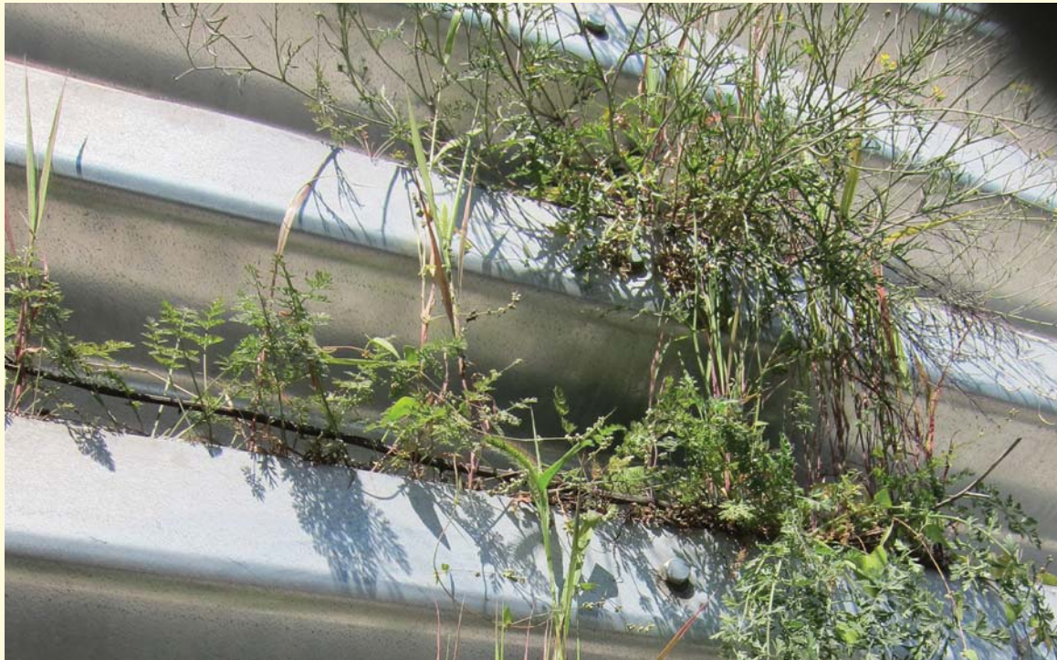
Figure 8.06: Colonisation of a steel wall by plants on a southern facing street-side retaining wall, Toronto.
