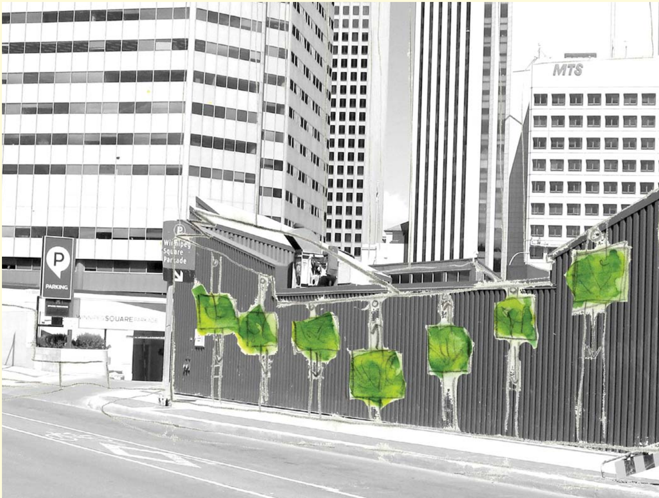
Figure 10.13: Gravity wall on Winnipeg Square.
