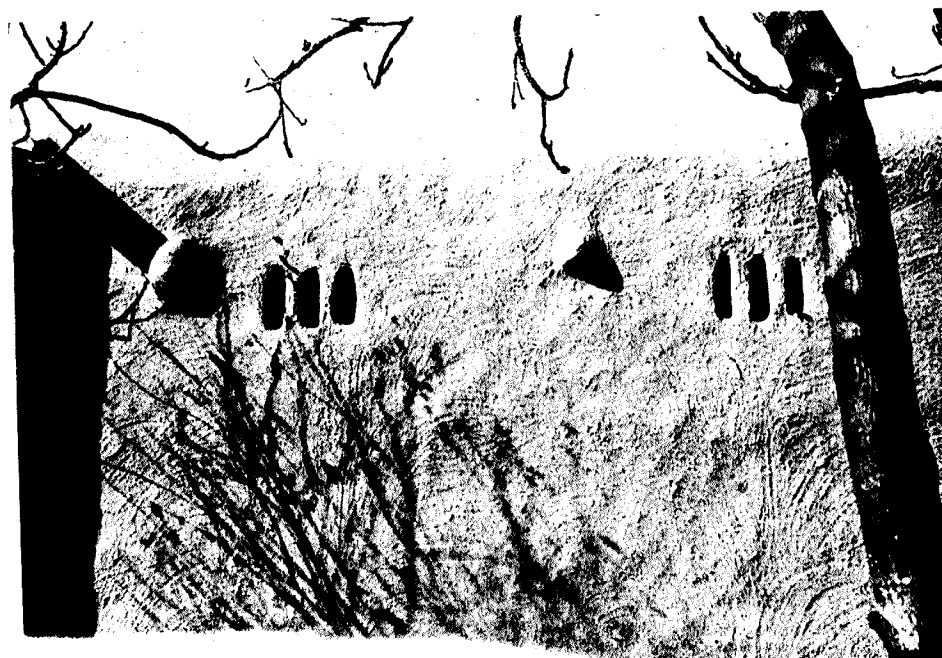
Openings in the wall
