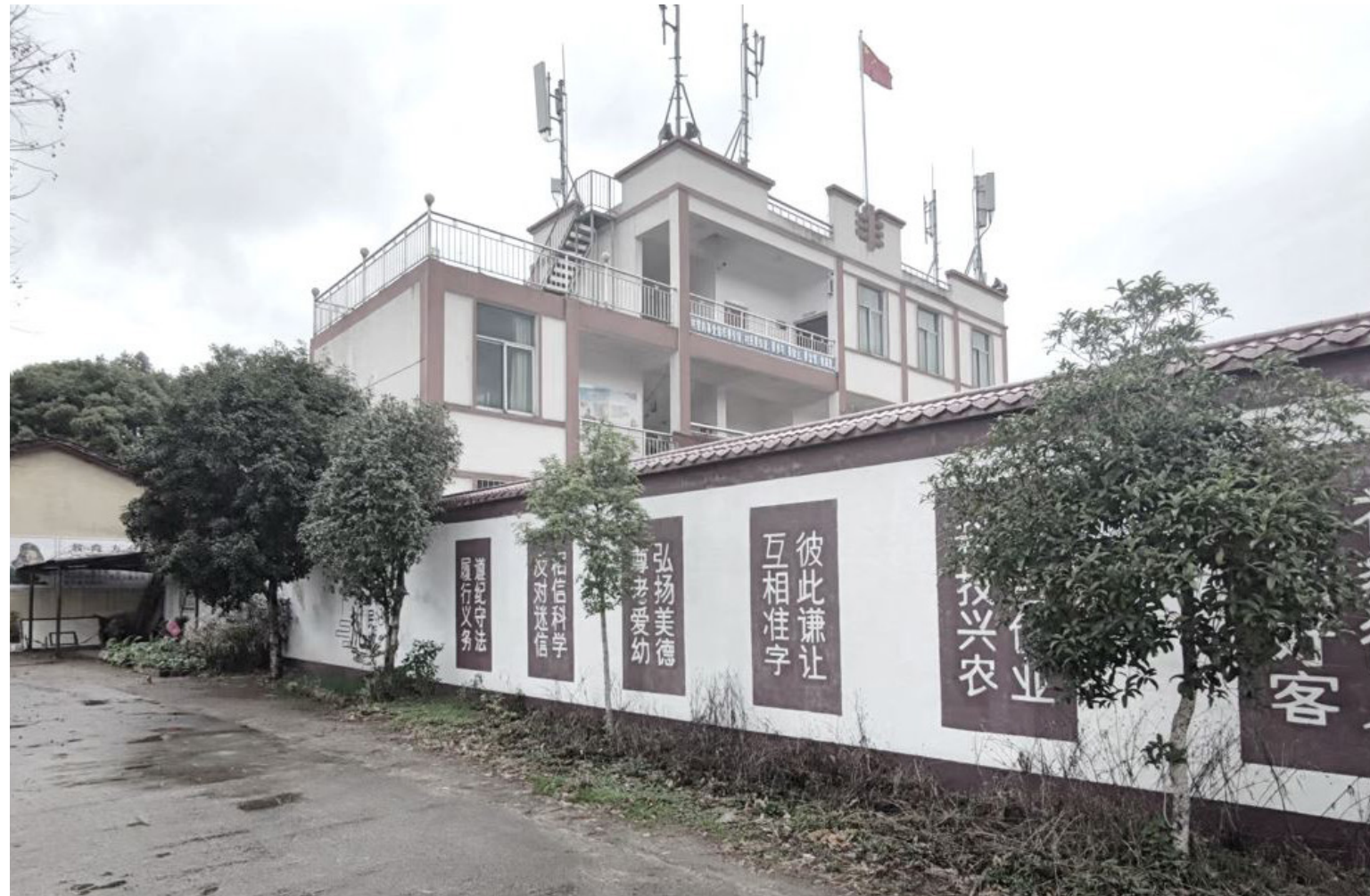
Figure 6-26: Existing condition of the community center
