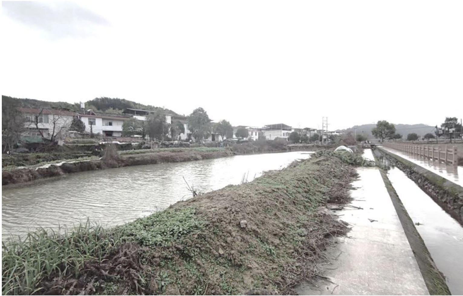
Figure 6-46: Existing condition of the pond
