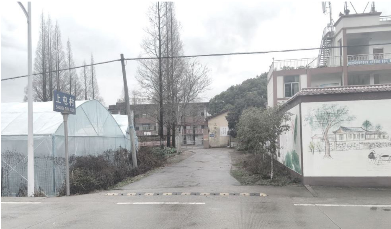
Figure 6-23: Existing condition of school entrance
