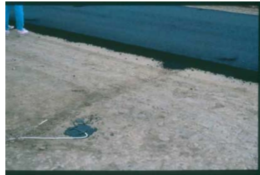
(b) Asphalt Strain Gauge Installation
