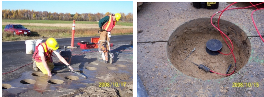
(a) Retrofit installation
