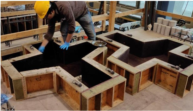
(A) Oiling Formwork before casting of concrete
