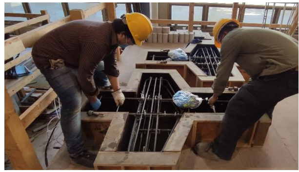
(B) Placing build reinforcement caging into the formwork.
