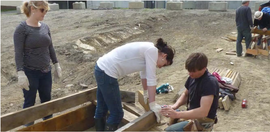
Fig. 6.3.2 Volunteers building planters. (Credit: Elaine Sedgman)
