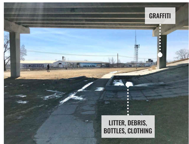
Fig. 7.3.16 Space under the overpass
