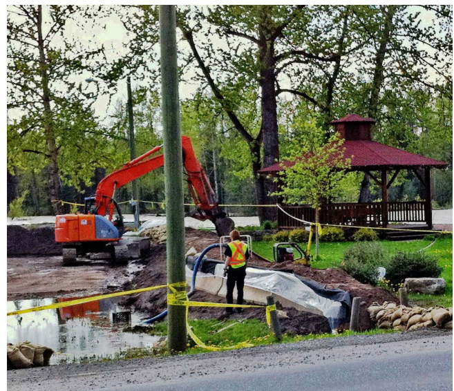
Fig. 8.7.4 Contracted construction work. (Credit: Province of British Columbia)
