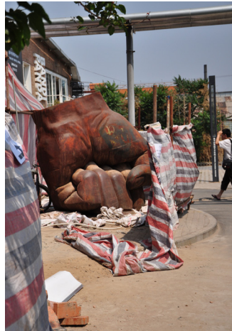
Figure 15: Public art under construction.
