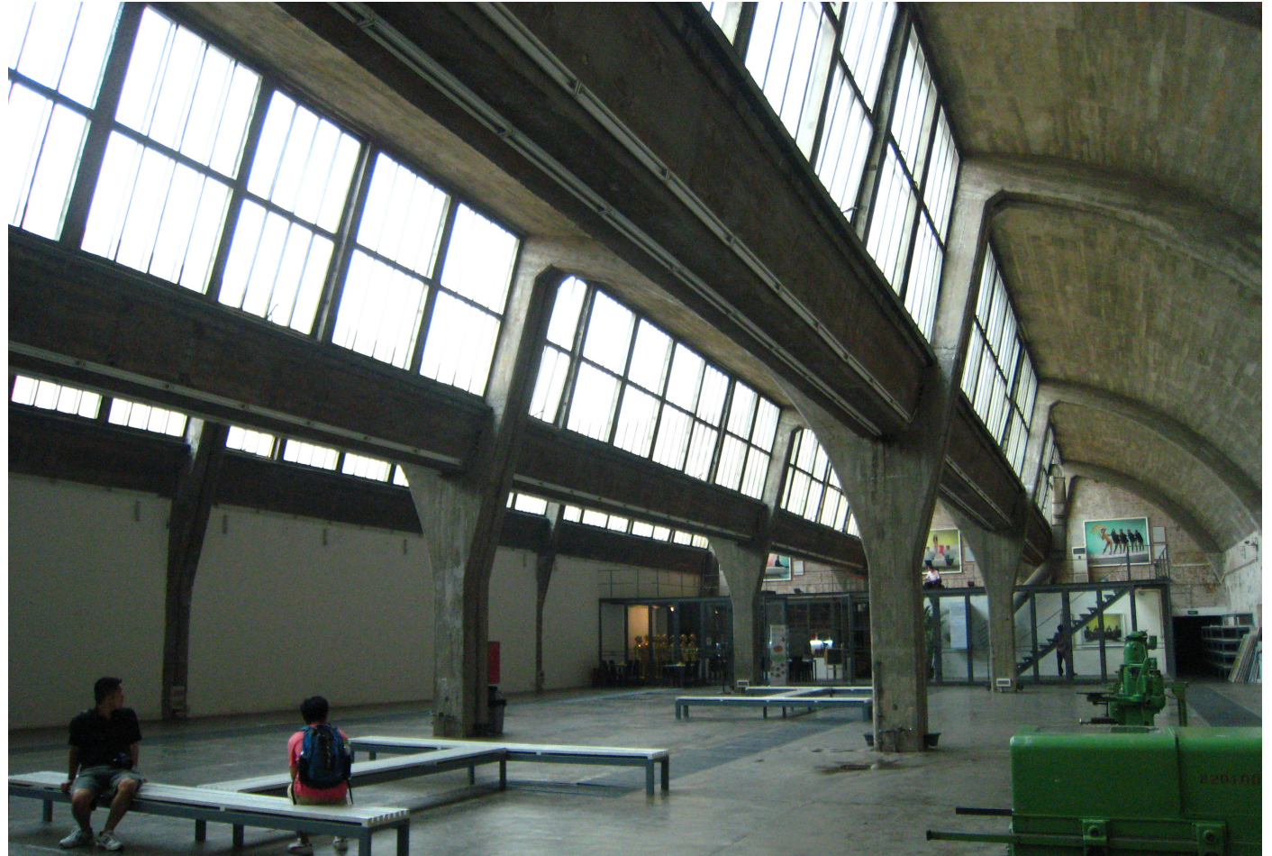
Figure 20: Sawtooth structure allows a soft diffused light to filter into Gallery 798 Space.
