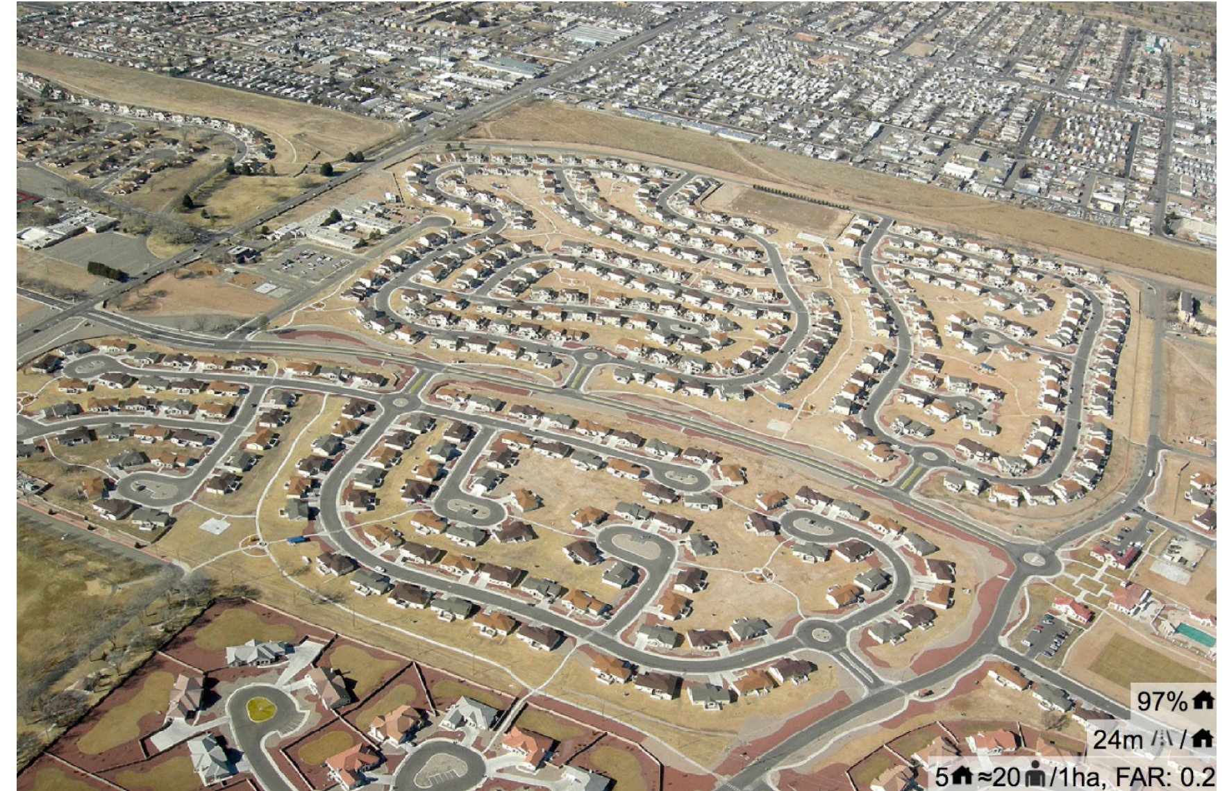
Figure 1.1 Subdivision urban sprawl in Albuquerque, New Mexico Photograph by Ivan Valiela, 2007. Used with permission from http://hermes.mbl.edu/news/features/images/aerial.jpg (accessed May 22, 2013)
