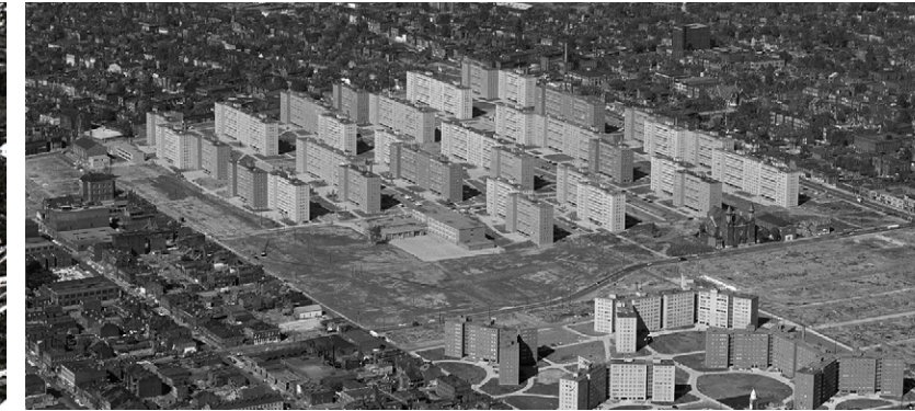
Figure 1.6 Pruitt-Igoe, St. Louis, Missouri, 1956-1970 Photo from United States Geological Survey. Public domain. Reproduced from http://en.wikipedia.org/wiki/Pruitt-Igoe#mediaviewer/File:Pruitt-igoeUSGS02.jpg (accessed August 10, 2013)
