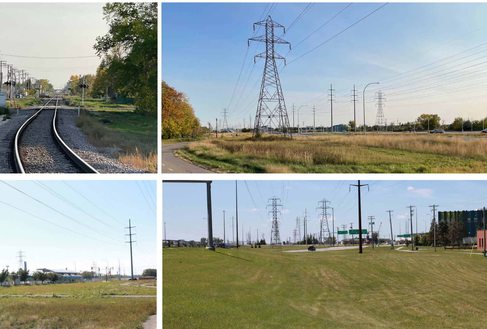
Figure 33: Site Investigations illustrating Existing Infrastructure Conditions
