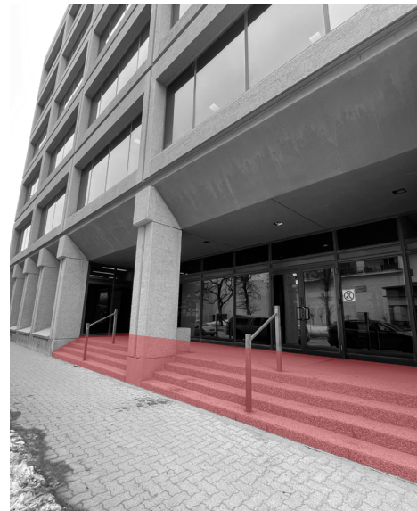
Non-accessible main entrance
