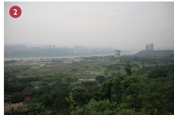
On the main access road looking south at the only remaining gas tower and the river. Such openness is rare in mountainous Chongqing.
