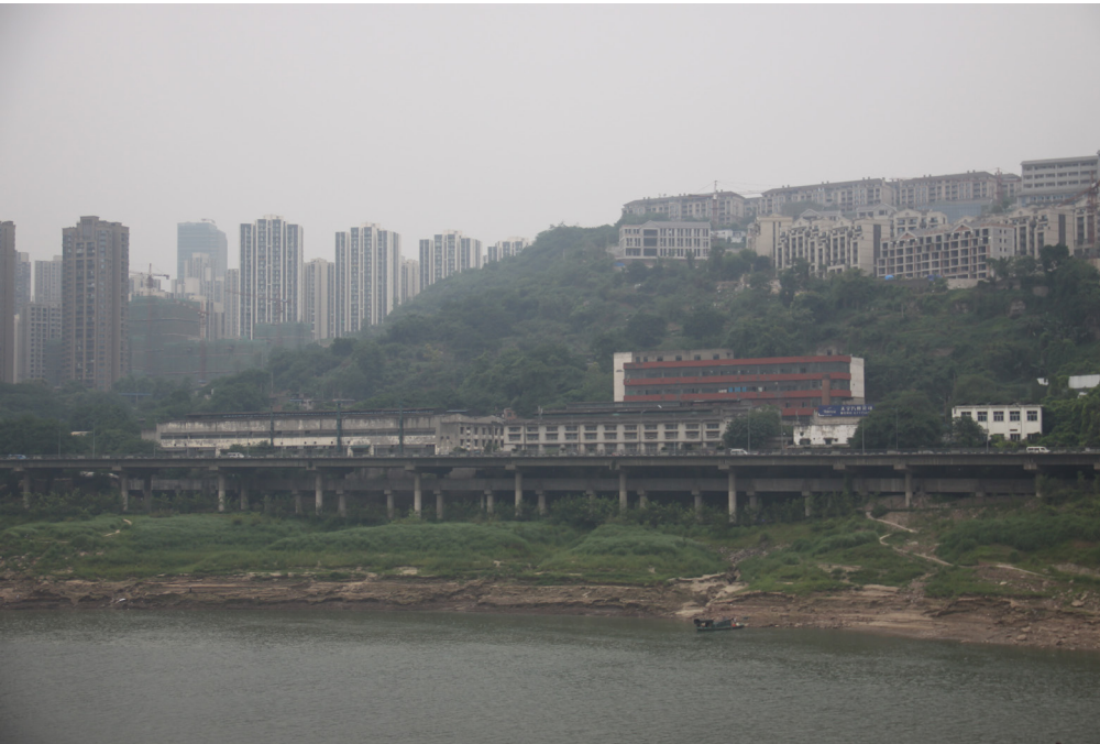
A decommissioned industrial military factory on the north bank of Jialing river,. The redevelopment plan has already been approved and will soon be underway.
