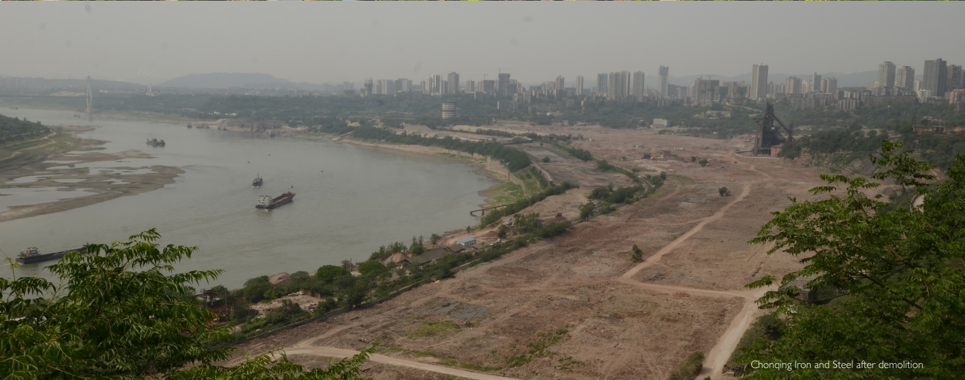
Chongqing Iron and Steel before demolition
