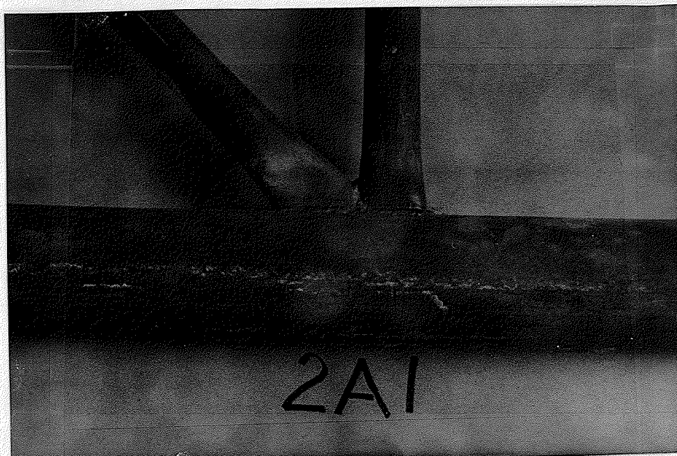
Photo 5.5 Joint 2A1 Detail
