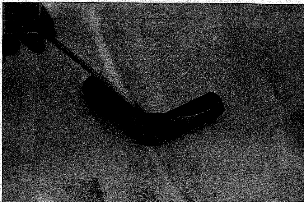
Photo 3.14 Crack In Seam Of Flattened H.S.S.
