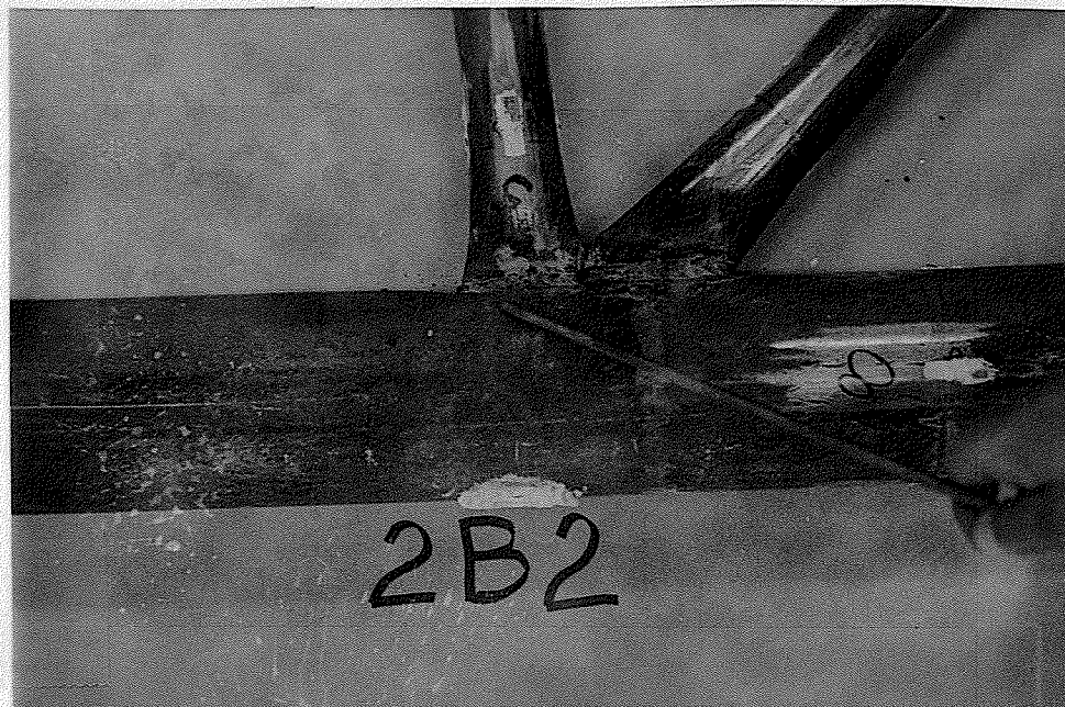
Photo 5.7 View Of Deformation Of Specimen 2B2 After Loading
