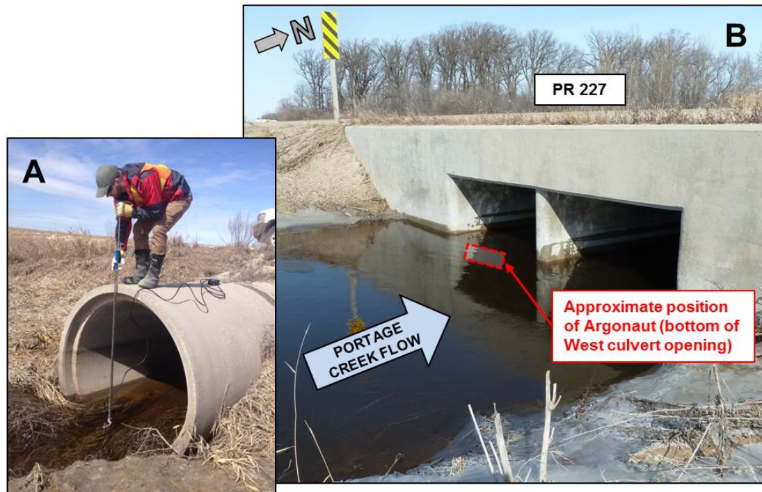
FIGURE 3.3: (A): Field measurement of point discharge with the FlowTracker at Station E2 (B): Site layout at Station E7
