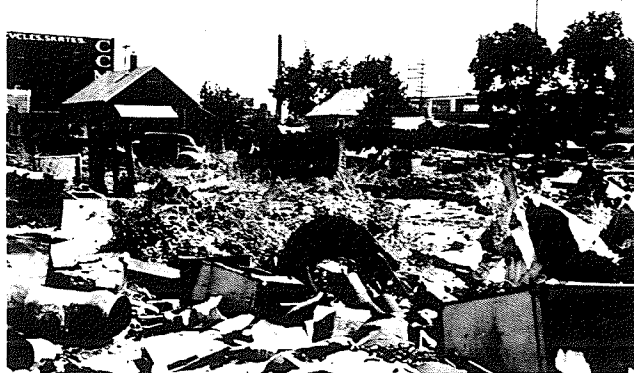
Debris on vacant lot
