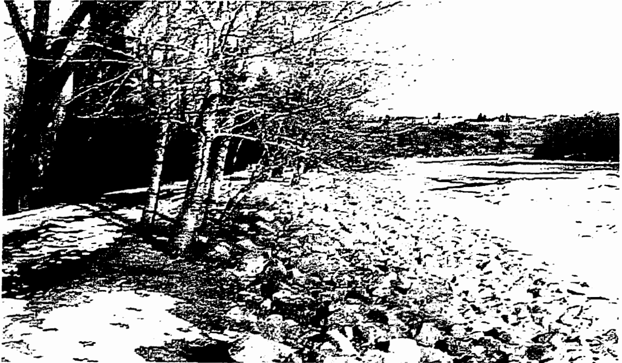
Figure 4.2a Rip Rap at the toe of a dike along the Bow River in Calgary
