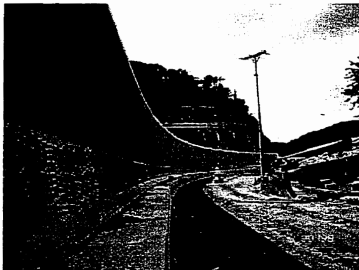
Figure 3.5.3b Large Concrete Flood Wall Source: U.S. Army Corps of Engineers
