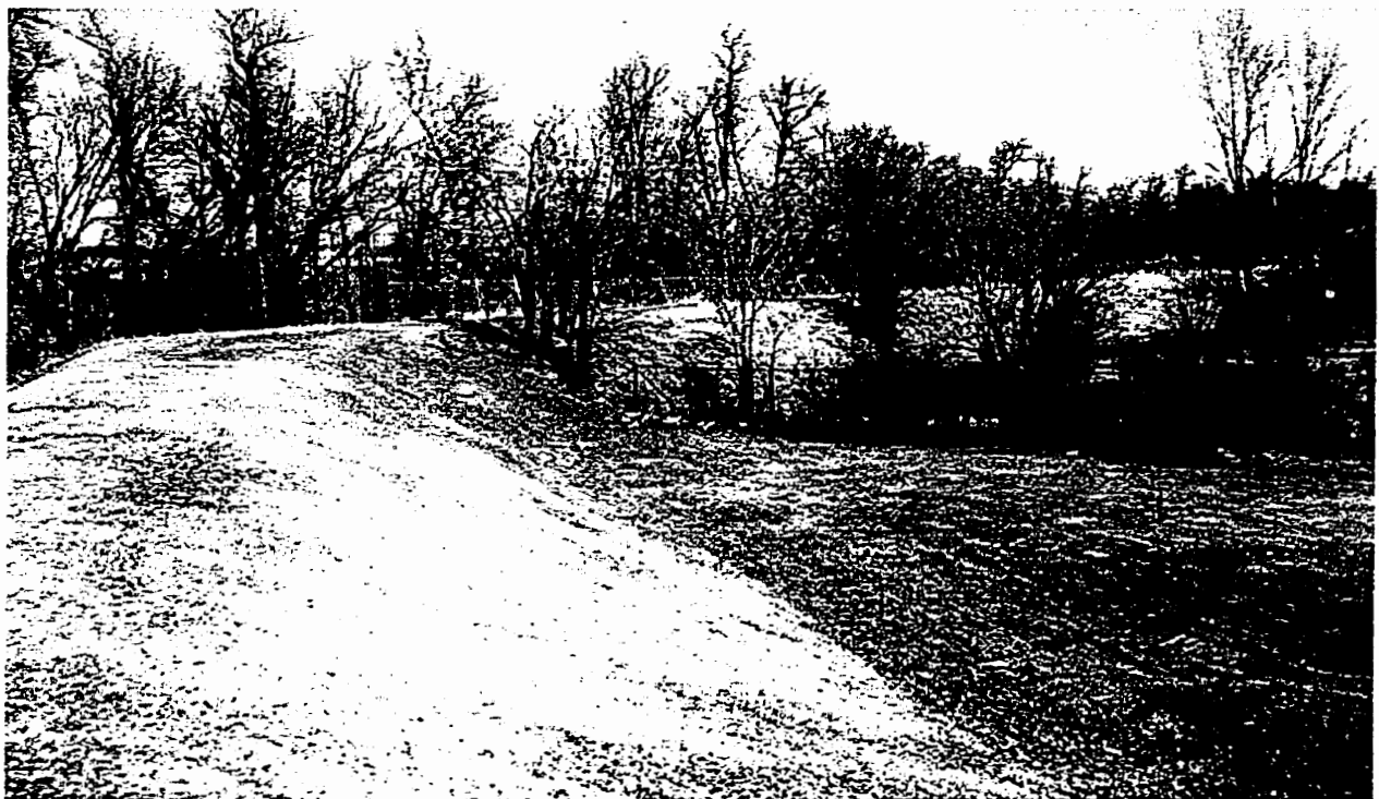
Figure 4.6 Typical grass covered dike
