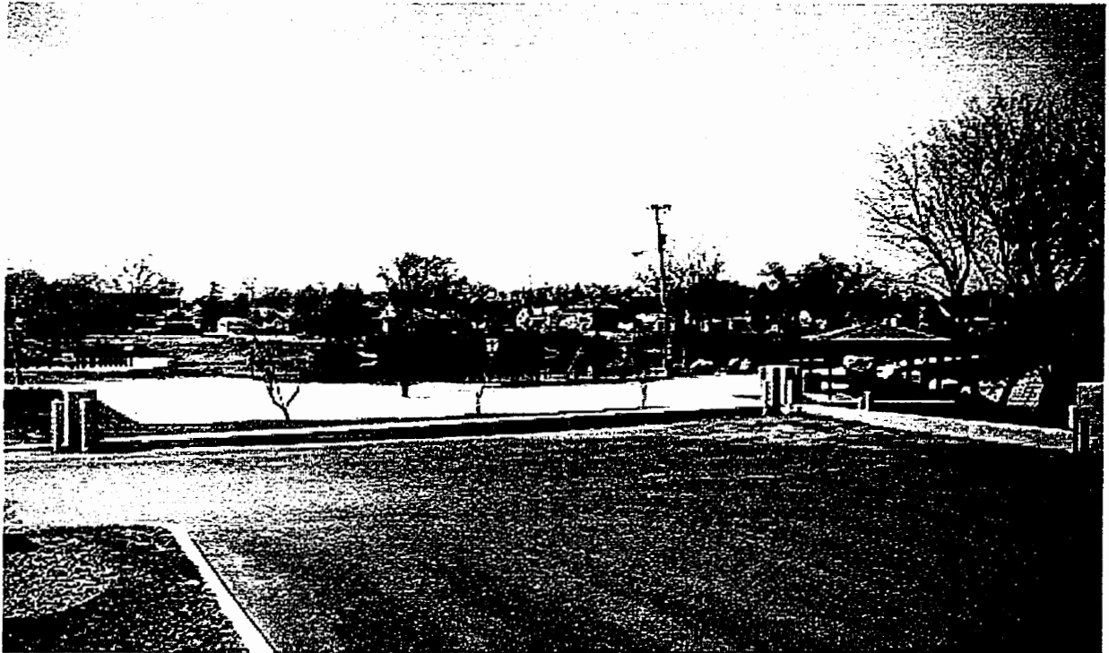
Figure 3.5.1c Minimal visual impact of permanent components of this floodwall Source: Flood Control of America
