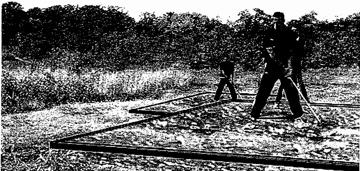
Figure 10.5d Tee boxes on extended dike crest
