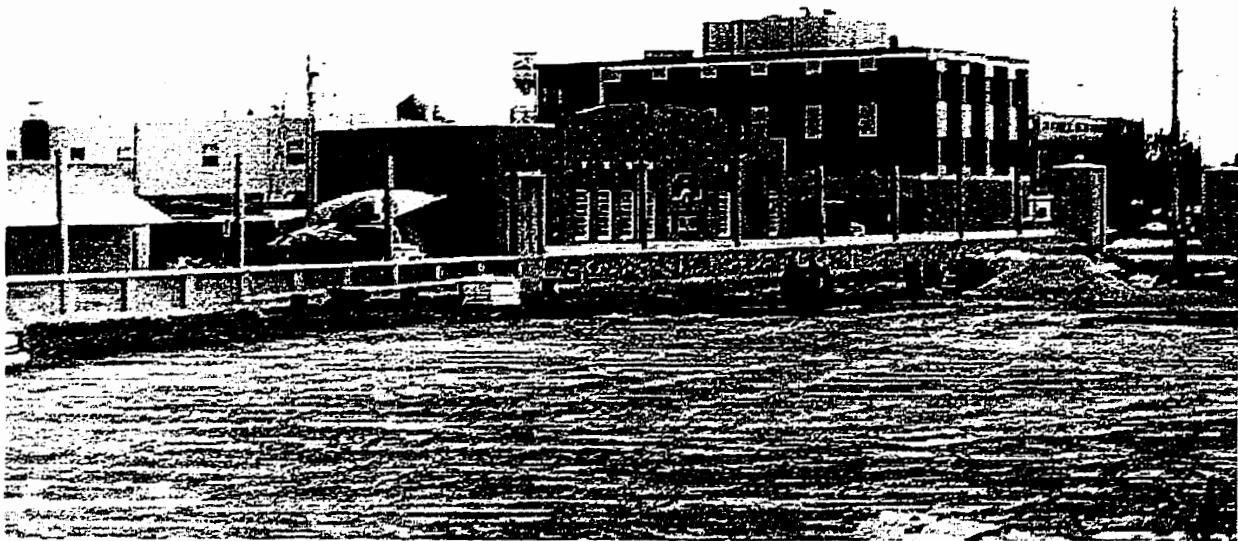
Figure 3.5.1h A new flood wall for the City of Grand Forks, North Dakota Source: Flood Control of America
