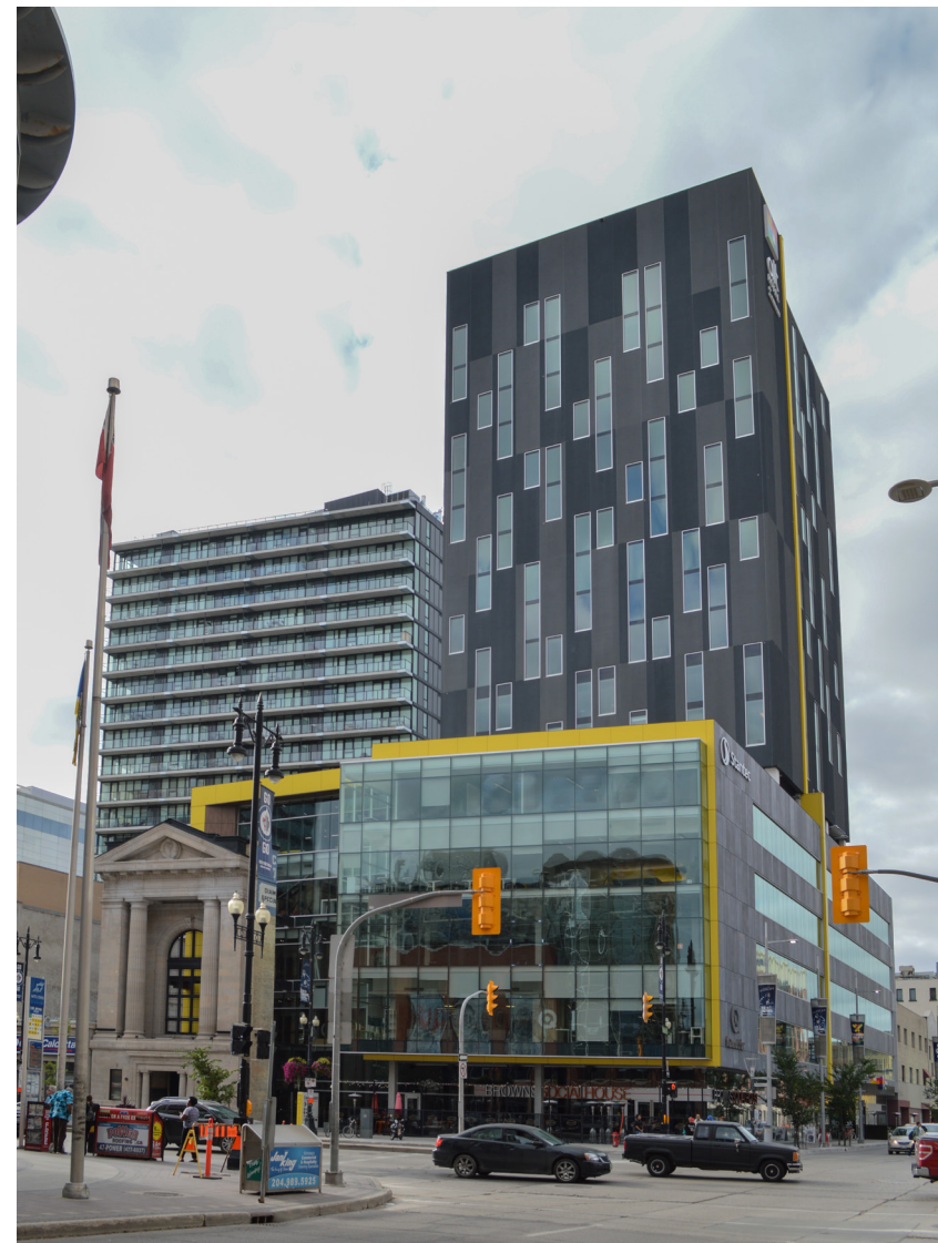
Figure 39. Photograph of the preserved Canadian Bank of Commerce facade in its current state, integrated into the south facade of Centrepoint.
