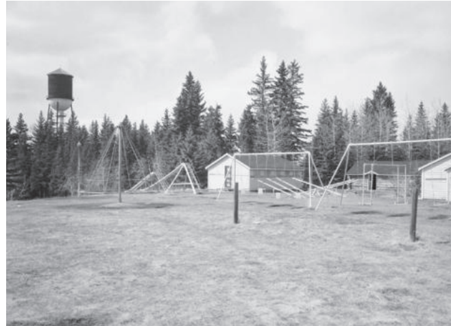
FIG. 1.6 The old 130 foot water tower and childrens' playground surrounded by spruce forest - Foto Arts Studio, 1955. Courtesy of Red Deer and District Archives. Used with permission
