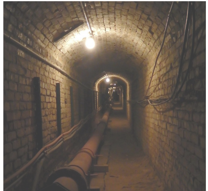
FIG. 5.10 "Steam tunnels (Grand Traverse Commons)" - Hathway, 2016
