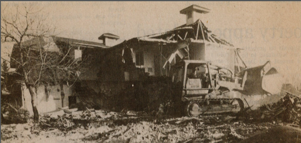
FIG. 1.13 Maple residence, built in the early 1930s, being demolished after a lifespan of approximately 50 years (1 of 7 slated for demolition in the 80s) - Red Deer Advocate, 1984. Used with permission
