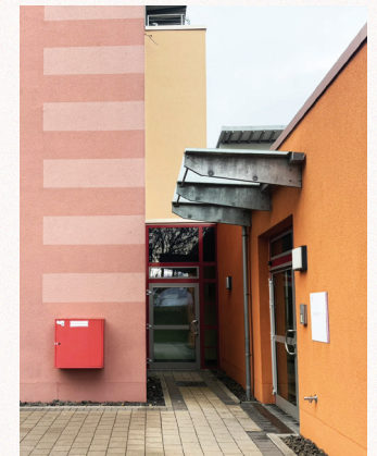
Fig 44. Fire escape entrance
