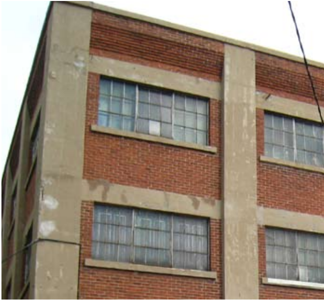
Figure 49 (above left) Detail of damaged windows and deterioration on facade
