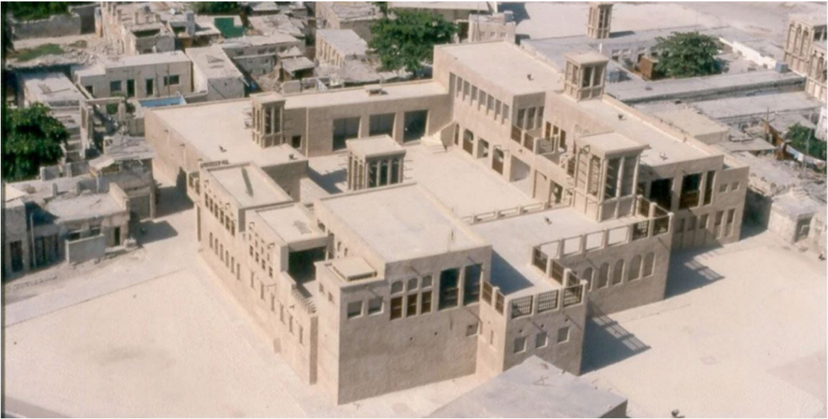
Fig.50 Aerial View of Sheikh Saeed Al Maktoum building
