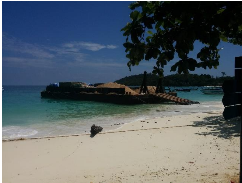
Figure 4.6: A platform on Pattaya Beach, Koh Lipe loaded with sand for construction
