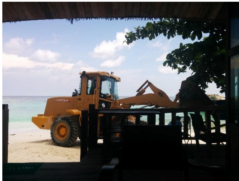
Figure 4.7: A tractor on Pattaya Beach transfers the sand from the platform to the construction site
