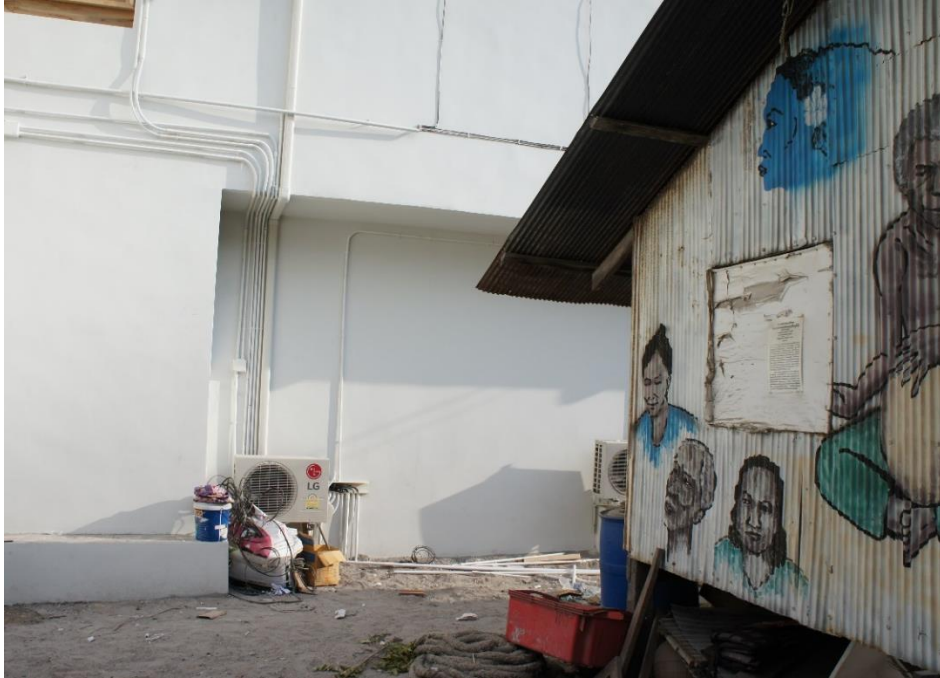
Figure 4.13: A large resort has been built adjacent to one of the Chao Ley villages near Sunrise Beach. The owners reported that they are constantly disturbed by resort workers and the air conditioners next to their home.
