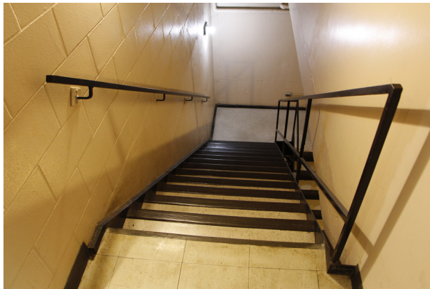
Figure 54: Stairs to Basement
