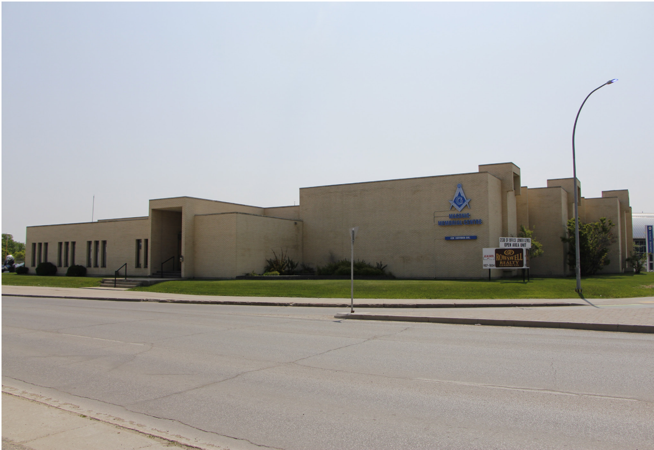
Figure 35: Masonic Memorial Centre – 420 Corydon Avenue, Winnipeg, MB
