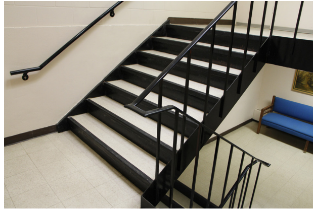
Figure 50: Stairs to basement
