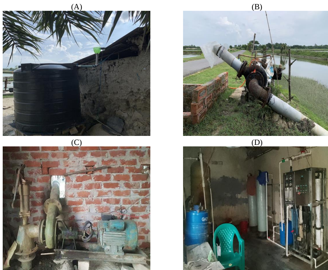
Figure 3.4 Technologies being used for water supply: (A) Rainwater harvesting (RWH) (B) Low-lifting pump (LLP) (C) Deep submersible pump (DSP) attached with deep tube well (DTW) (D) Reverse osmosis plant (RO).
