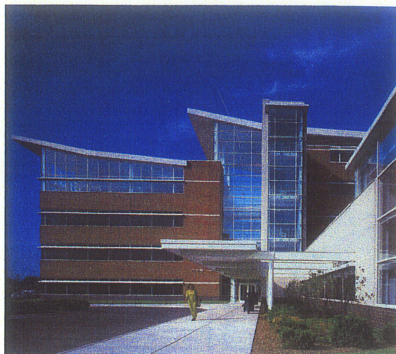
Figure 7: Exterior Entrance – CORE AIDS Center
