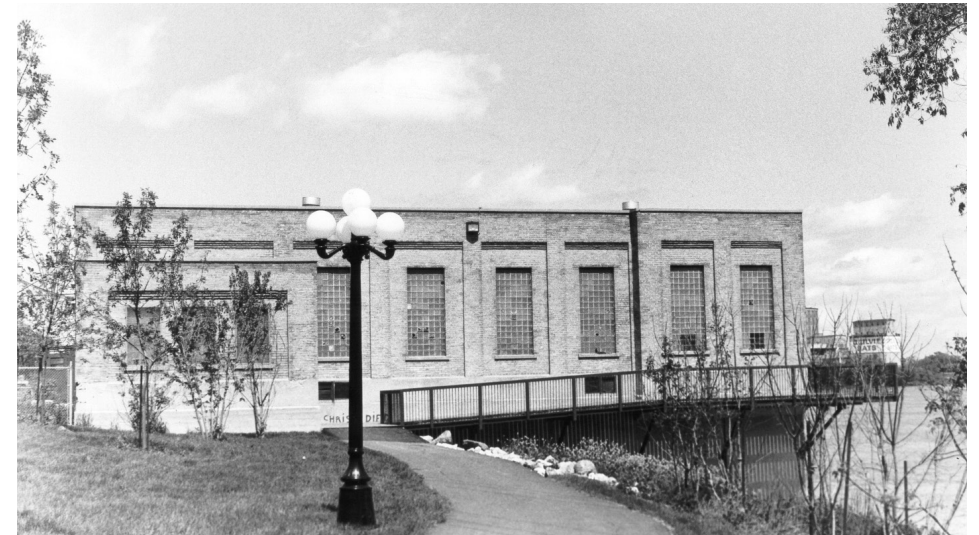
▲ F68 | PEDESTRIAN WALKWAY
