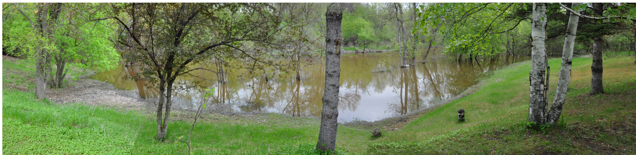
▼ F24 | JOCELYN HOUSE HOSPICE | RIVERBANK EROSION
