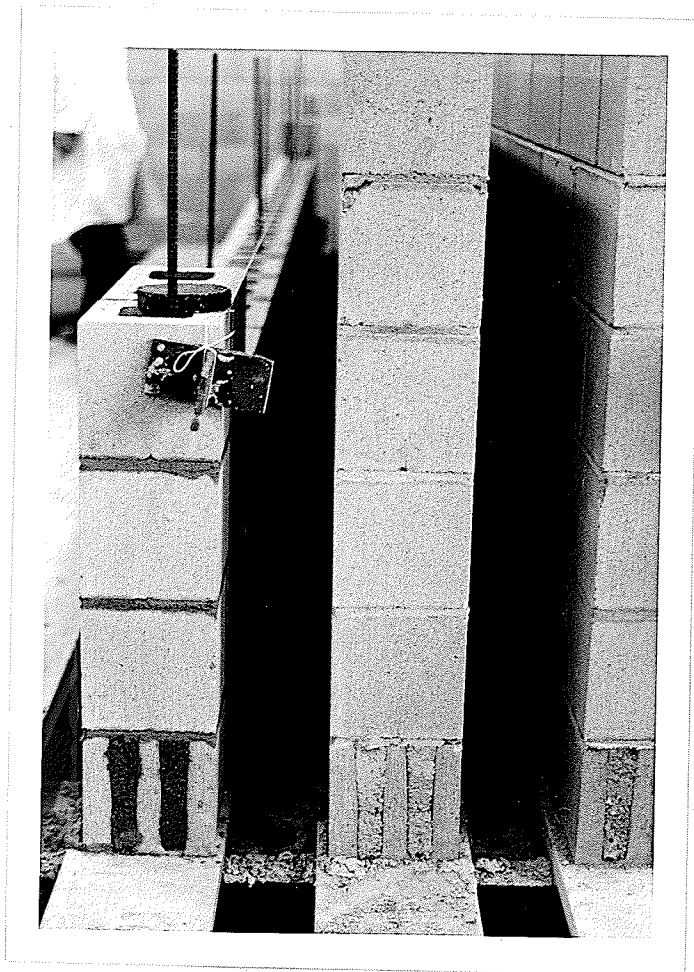
FIG. 11 ALIGNMENT OF HORIZONTAL GUIDE LINE
