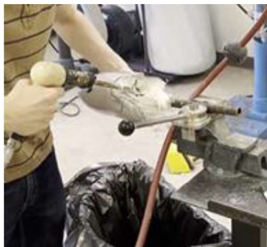
Figure A12 - Air chisel removing plaster
