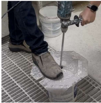
Figure A4 - Mixing plaster mix
