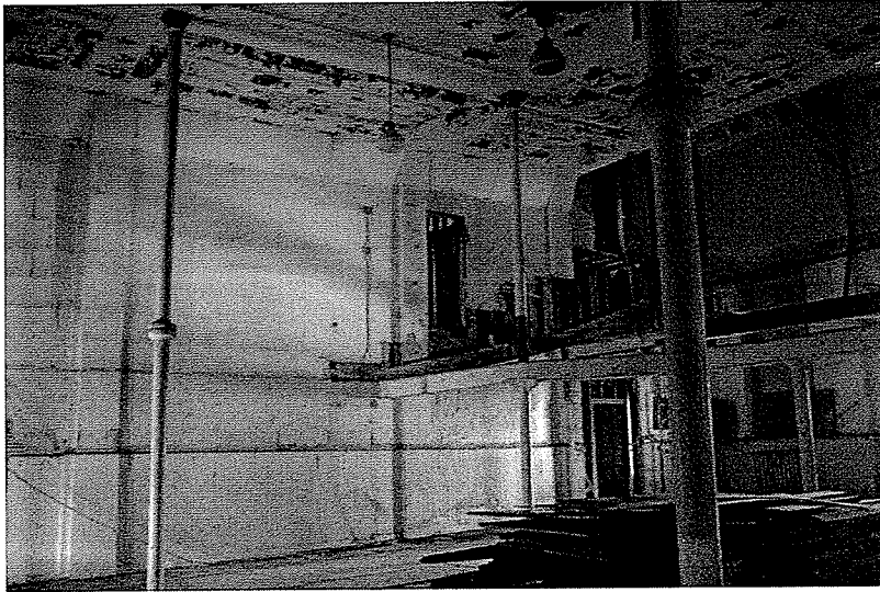
Figure 6.10 Salvation Army Citadel, Winnipeg, Manitoba, 2004. Traces outlined on third level North and South walls indicate stepped segments of the original gallery. Photograph by Brianne Caron.
