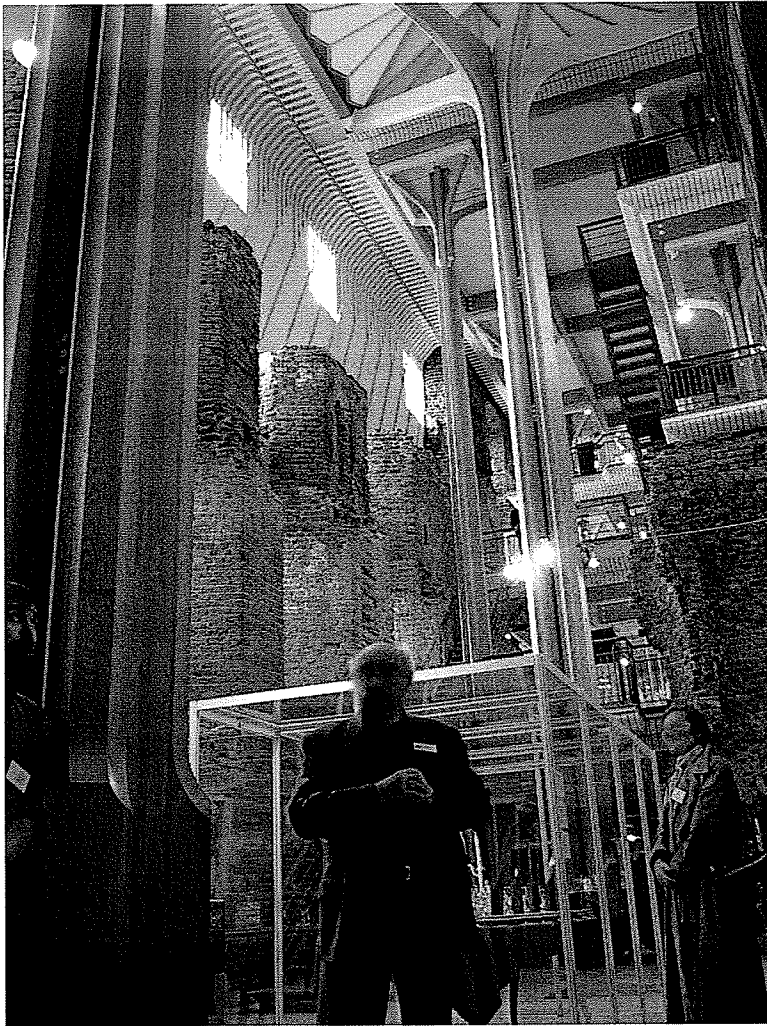
Figure 2.2 Koldinghus Castle, Kolding, Denmark, 13 th century commission. Restoration from 1972-1994 by Inger and Johannes Exner. Freestanding columns support a timber roof structure, inserted within the ruin. Photograph by James N. Weatherall. Courtesy James N. Weatherall.
