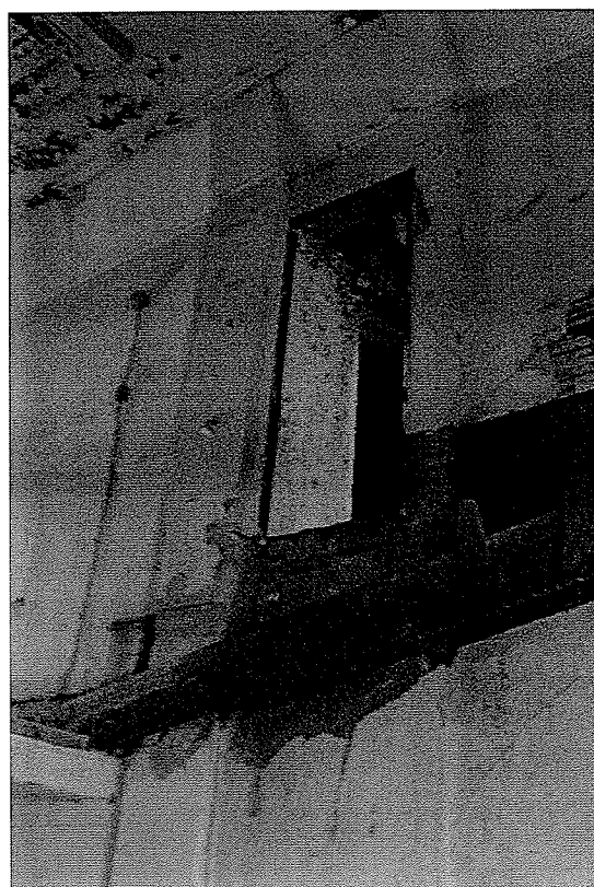
Figure 6.9 Salvation Army Citadel, Winnipeg, Manitoba, 2004. Traces outlined on third level North and South walls indicate stepped segments of the original gallery. Photograph by Brianne Caron.
