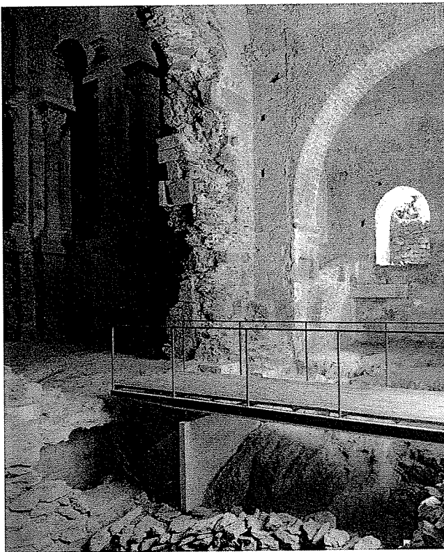
Figure 4.8 Sant Pere de Rodes, Port de la Selva, Catalonia, Spain. Intervention, 1993, Jose Antonio Martinez Lapena and Elias Torres Tur. Wood bridge on concrete pillars is suspended over significant archaeological excavations. Photograph by Hisao Suzuki. Courtesy El Croquis Editorial.
