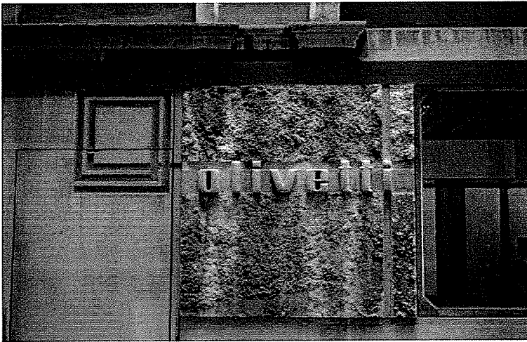
Figure 3.5 Olivetti showroom, Venice, Italy. Intervention, 1957-58, Carlo Scarpa. The Olivetti façade is detailed in order to accept and anticipate weathering in time. Photograph by Jonas Lehrman. Courtesy Jonas Lehrman.
