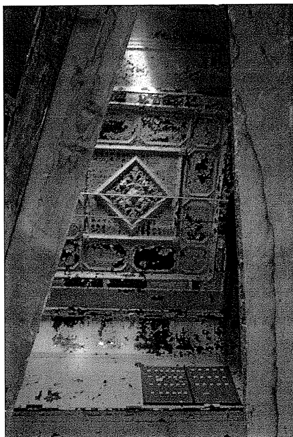
Figure 8.1 Salvation Army Citadel, Winnipeg, Manitoba, 2004. Pressed tin ceiling pattern defines the auditorium sanctuary ceiling. Photograph by Brianne Caron.
