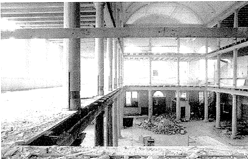
Figure 7.1 Trust Theatre, Amsterdam, 1793. Intervention, 1995, Mecanoo Architects. View of church interior prior to design intervention; a double colonnade of wood Tuscan columns forms the church interior. Photograph by Francine Houben. Courtesy Mecanoo Architects.
