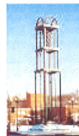
Above: the belltower at the corner of Stradbrook Avenue and Osborne Street serves as a distant landmark.
