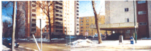
Above: Apartments in the Roslyn Crescent area. Massive scale, cul-de-sacs and fewer trees contribute in making this a distinct district.
