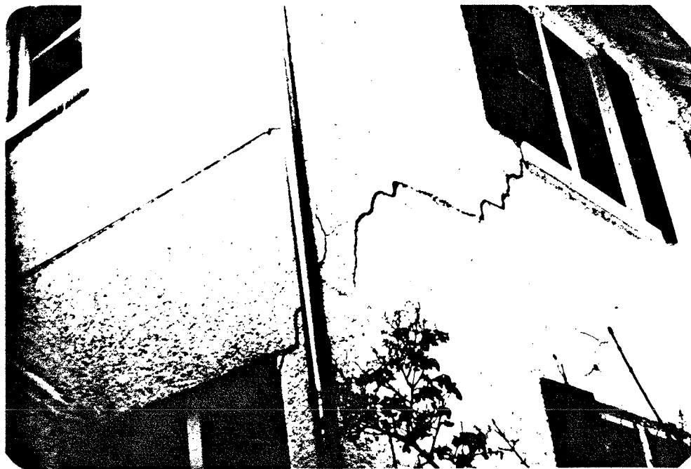
Figure 28 Cracks in Exterior Walls
