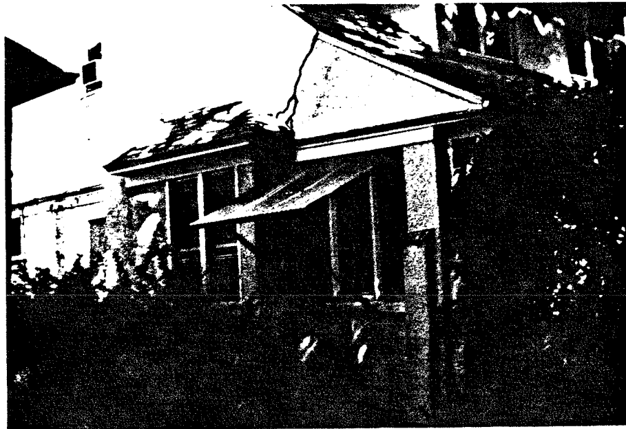
Figure 32 Differential Settlement of Additions
