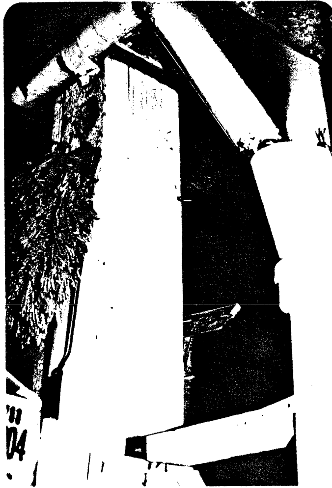
Figure 31 Separation Between Main Beam and Wooden Post
