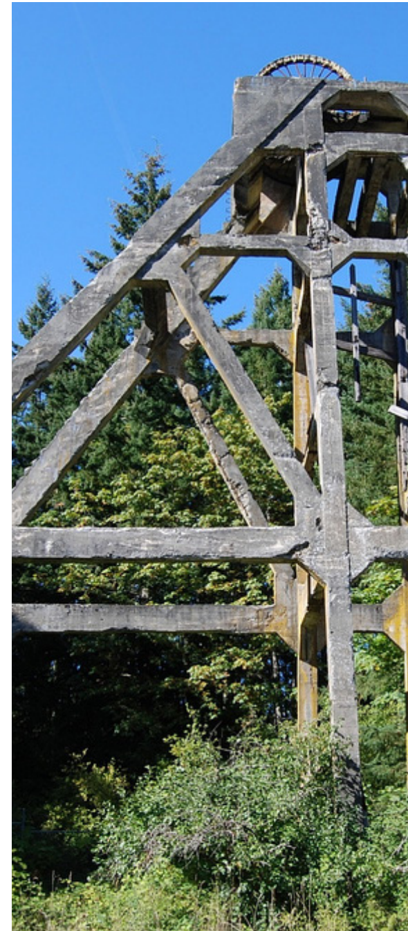
fig.53 Concrete ruin at Morden mine site 2012.
