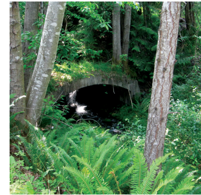
fig.114 Mine shaft entrance in Extension 2011.
