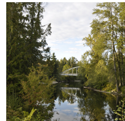
fig.80 Existing vehicle bridge across the Nanaimo River 1 km north of Origin Island
