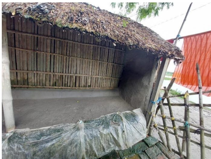
Note: Plastic covering edges and walls of mud houses to prevent salinity in the atmosphere from eroding the material
